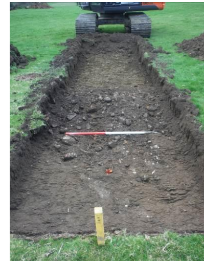
Trench 2: Stone dump (223), looking SW, 1m scale in 50cm divisions
