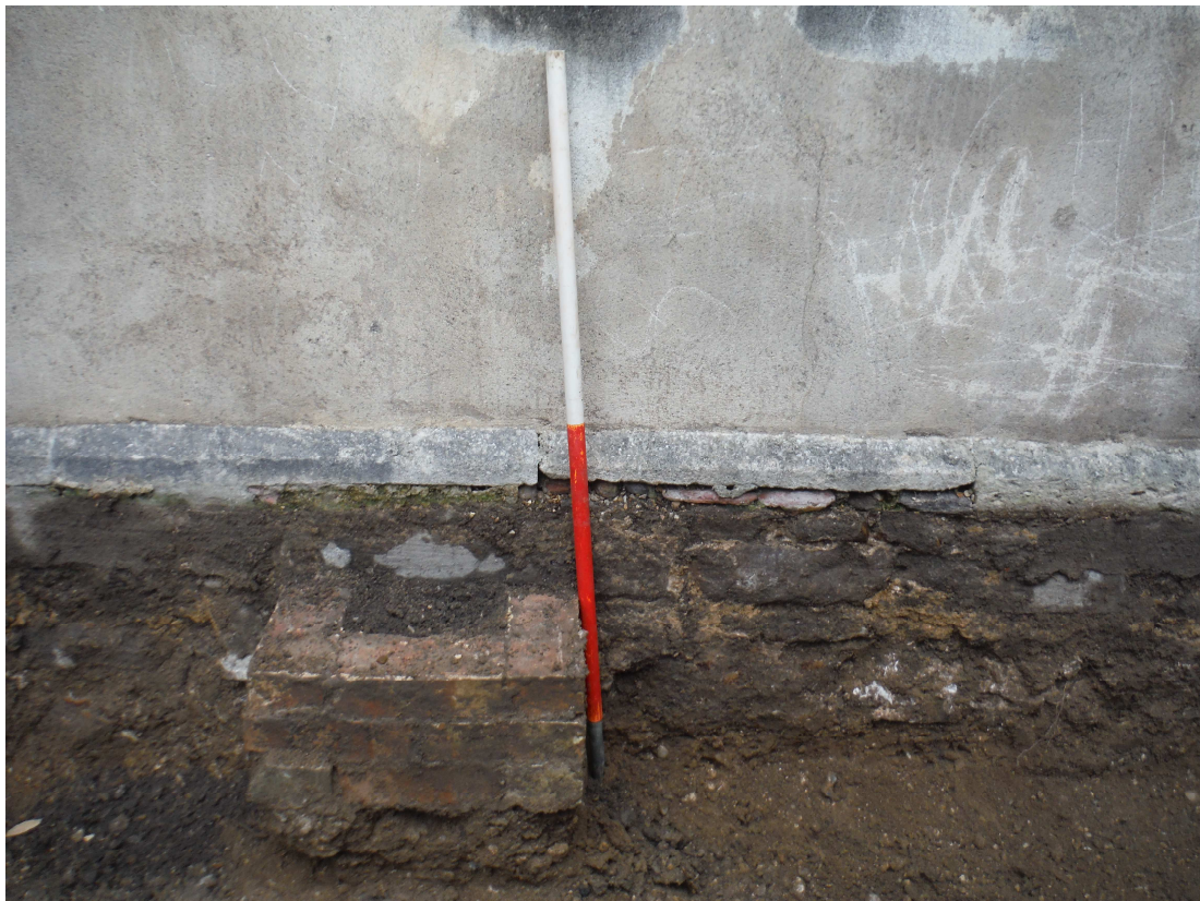
Plate 2: Trench 1 – nave foundation, south side, looking north (1m scale)
