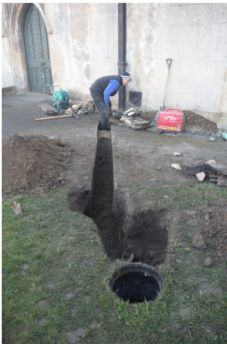
Plate 5: Trench 4 – looking south-east towards north-west corner of chancel
