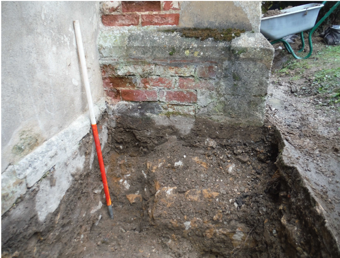
Plate 1: Trench 1 – pilaster buttress foundation, looking east (1m scale)
