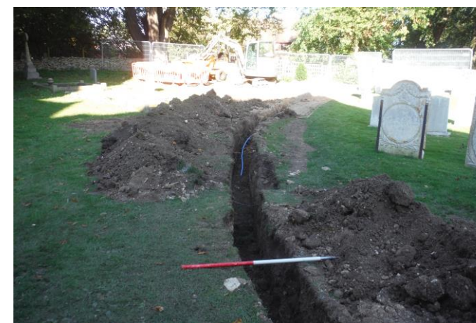
Plate 3: Trench 2 – general shot, looking NE (scale 1m)
