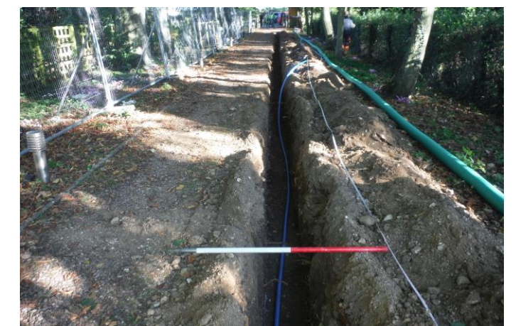
Plate 4: Trench 3 general shot, looking ESE (scale 1m)
