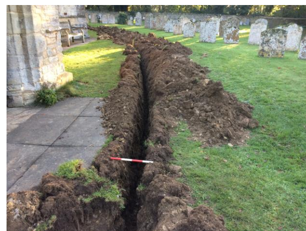
Plate 2: Trench 1 – general shot, looking east (scale 40cm)
