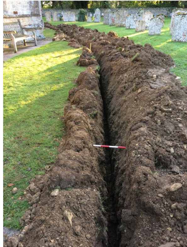
Plate 5: Trench 1 – general shot, looking NE (scale 40cm)
