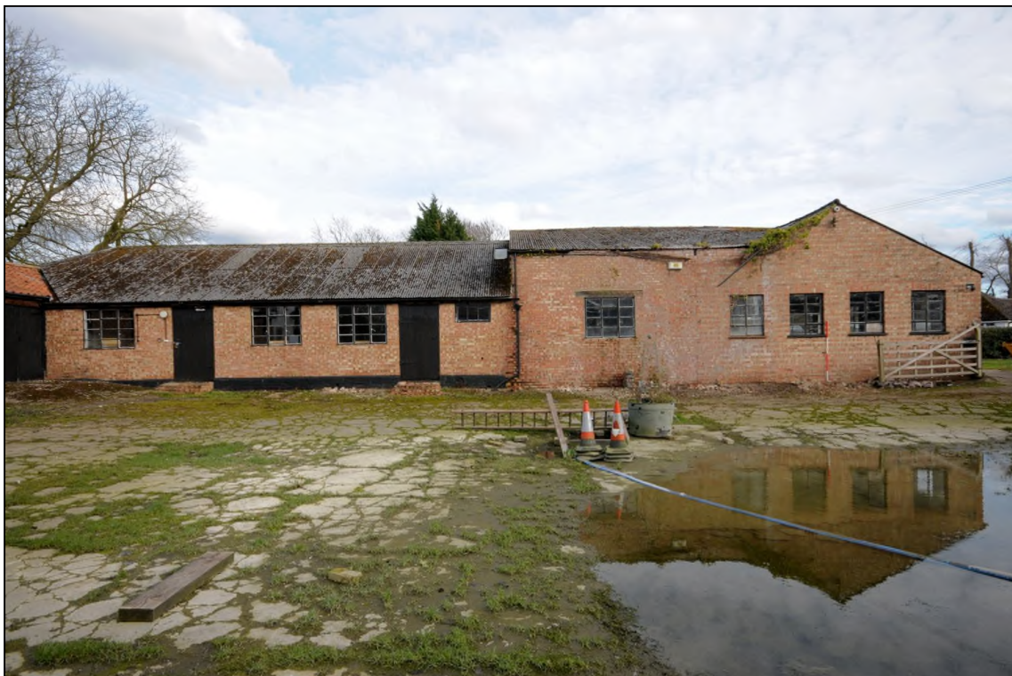
Image 2: West elevation of the workshop
