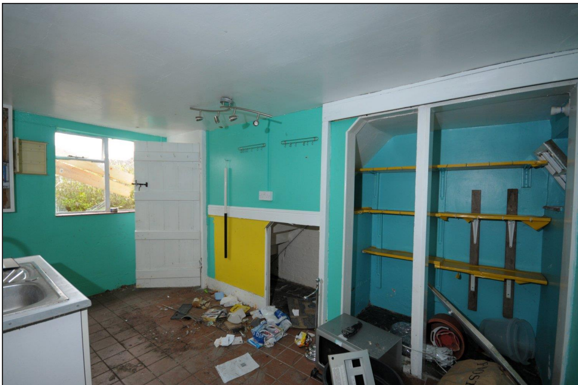
Image 34: No. 43, kitchen, looking south-east
