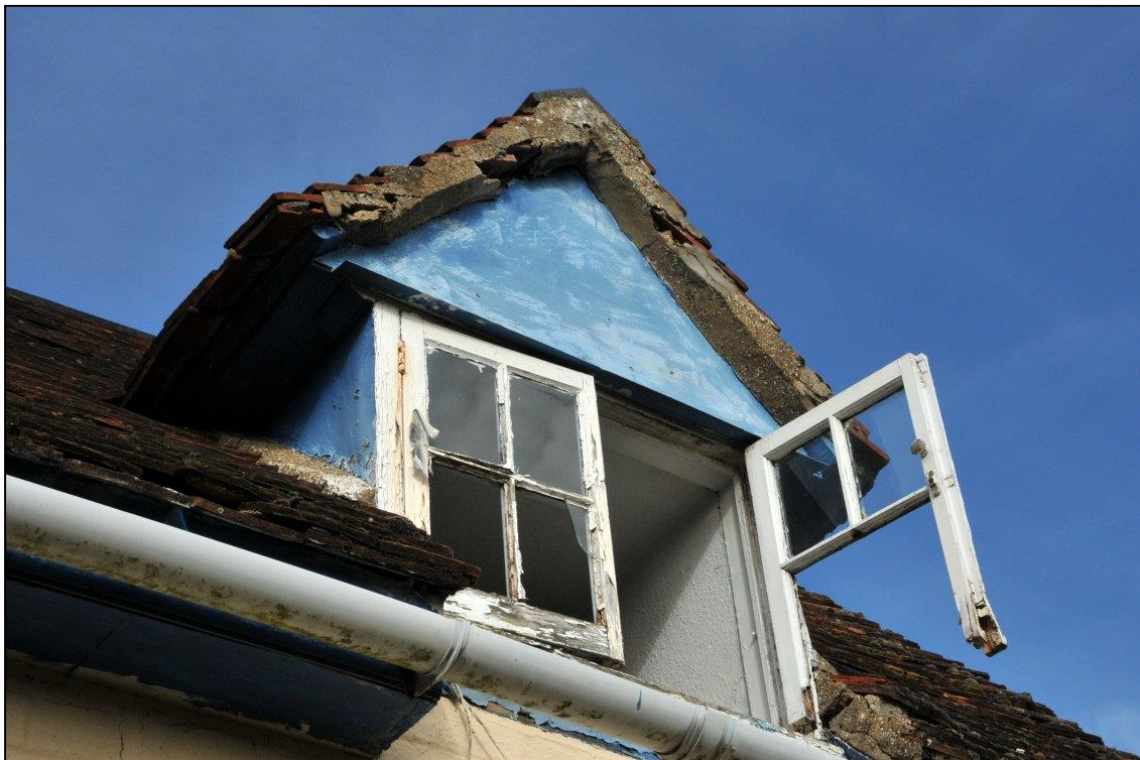
Image 4: South elevation, detail of dormer window
