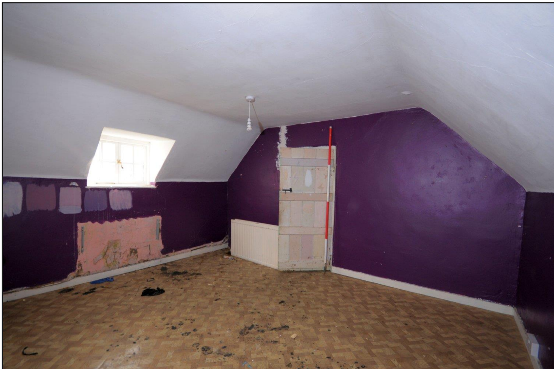
Image 24: No. 41, bedroom 1, looking south-east
