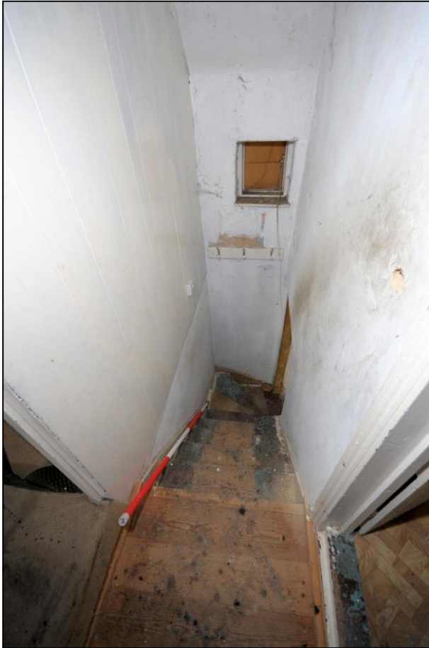
Image 23: No. 41, stairs and landing
