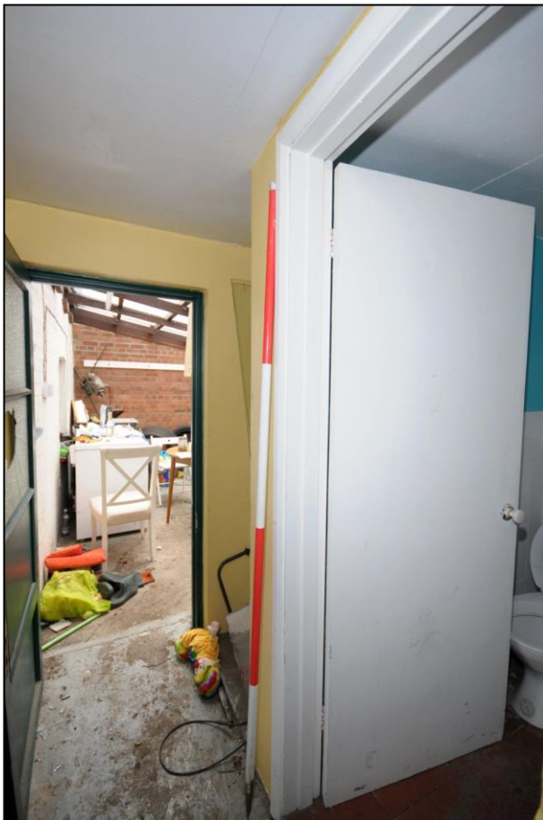
Image 38: No. 43, rear extension Looking south towards the conservatory (Scale 2m)
