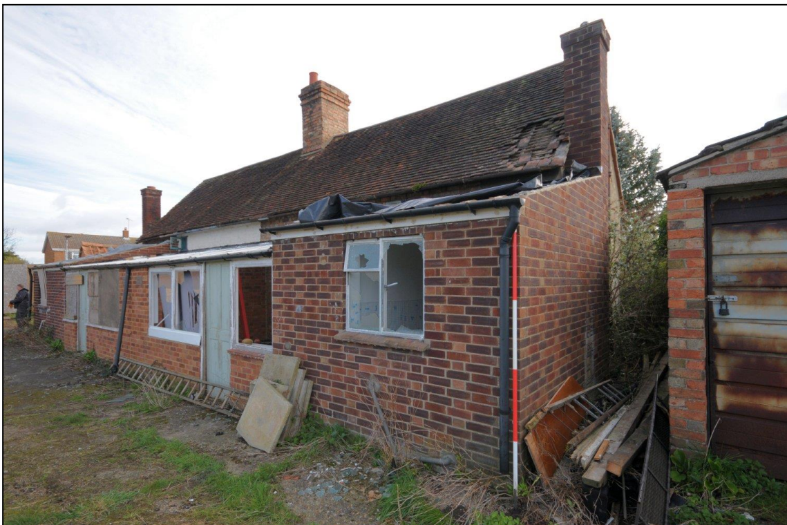
Image 8: Rear elevation, viewed from south-west
