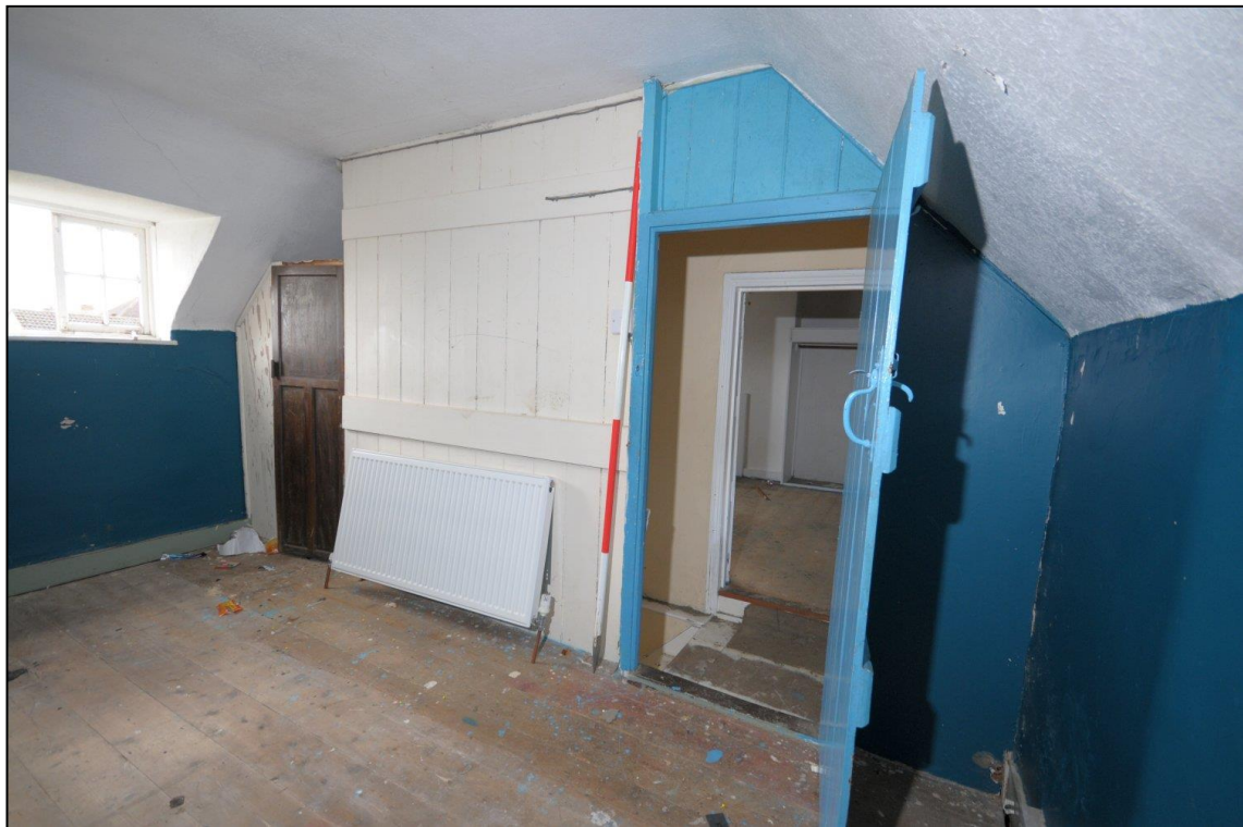
Image 48: No. 43, bedroom 2, looking south-east Boarded partition enclosing north side of stairs (Scale 2m)
