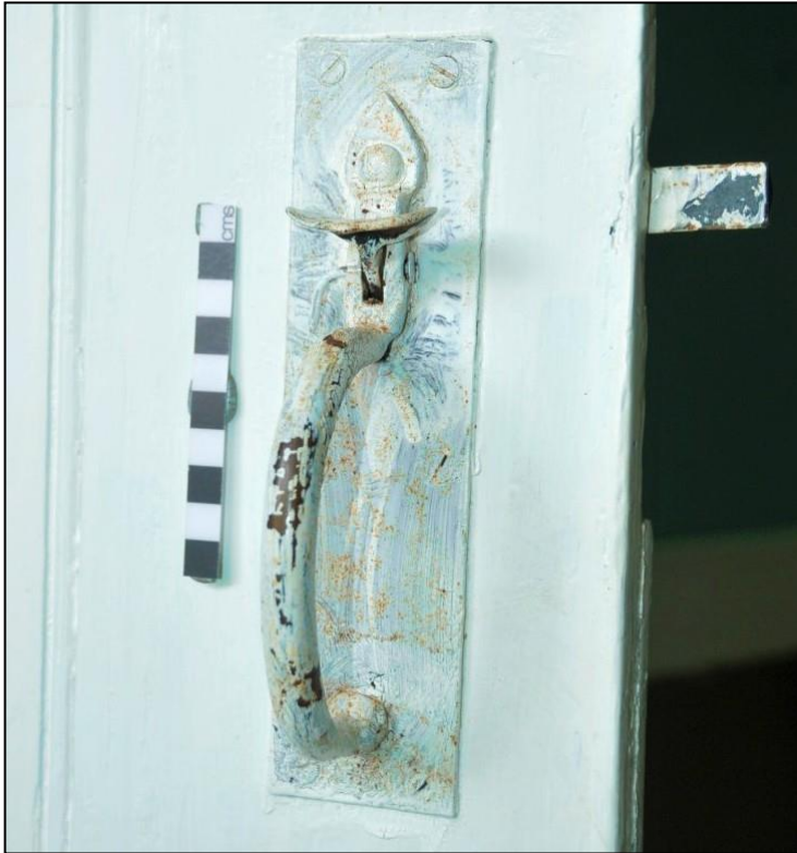
Image 37: No. 43, kitchen, door latch (Scale 10cm)
