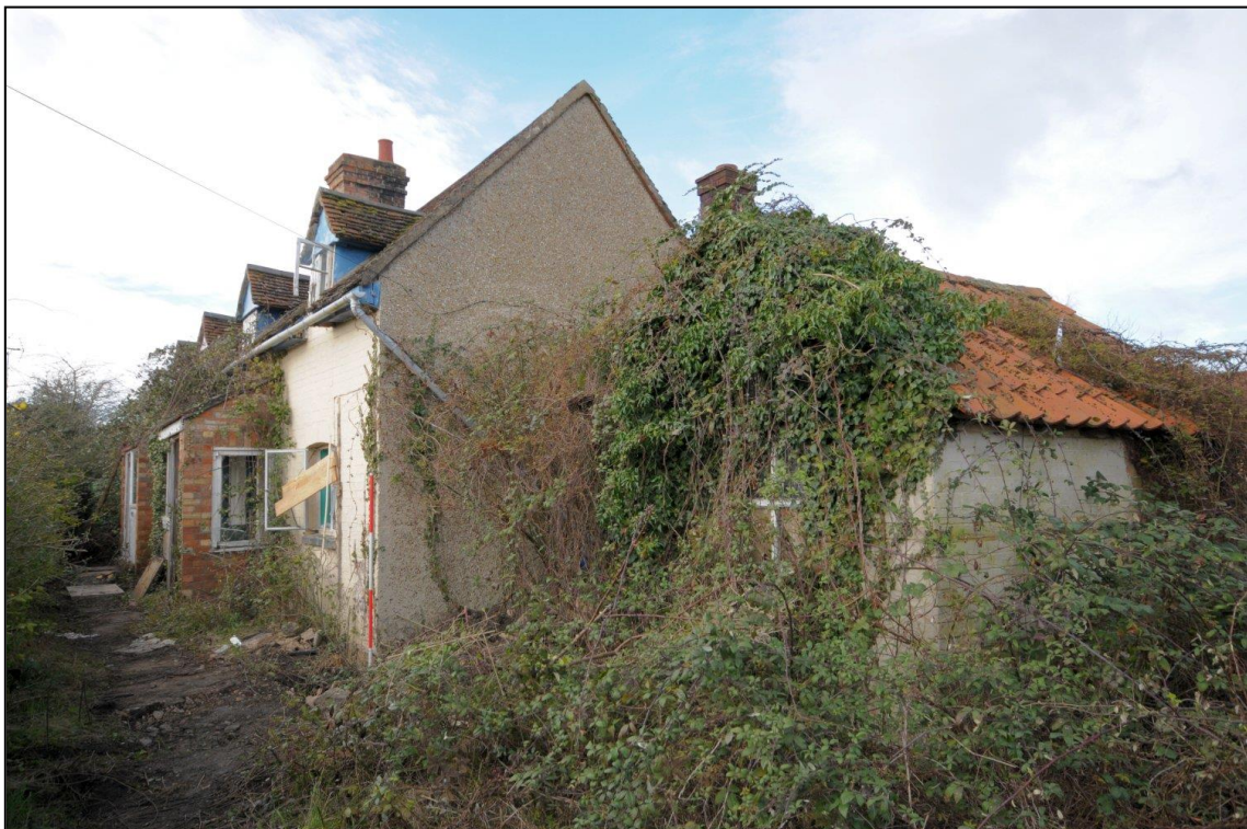
Image 2: North elevation North end of No. 43 with its shed to the right
