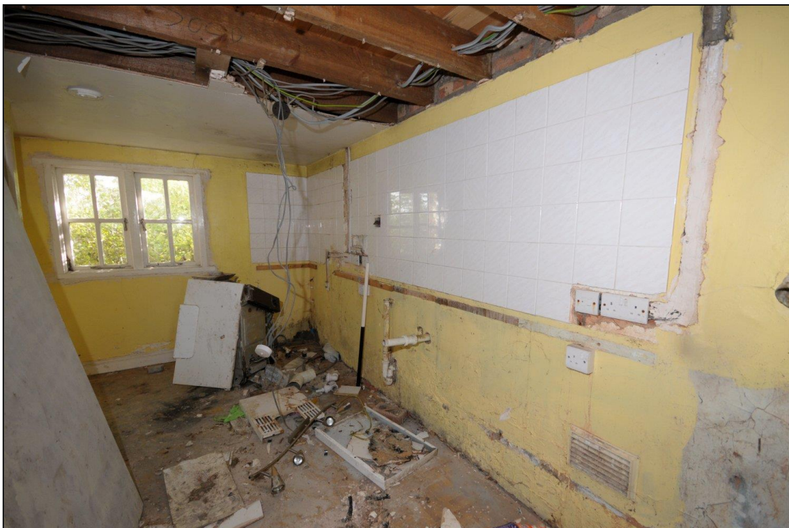
Image 15: No. 41, kitchen, looking south-east
