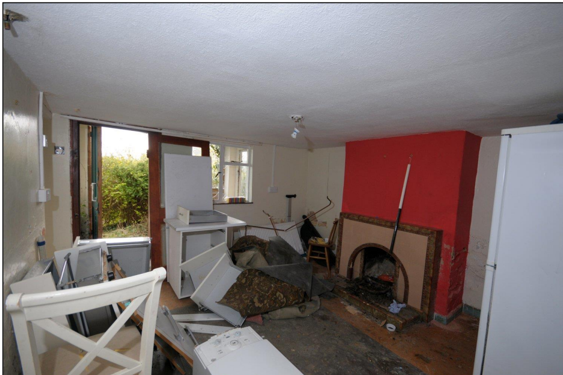
Image 30: No. 43, living room, looking south-east
