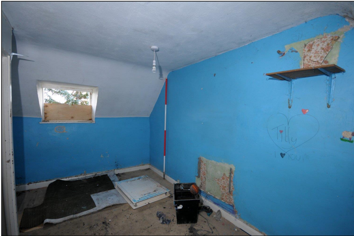
Image 29: No. 41, bedroom 2, looking south-east
