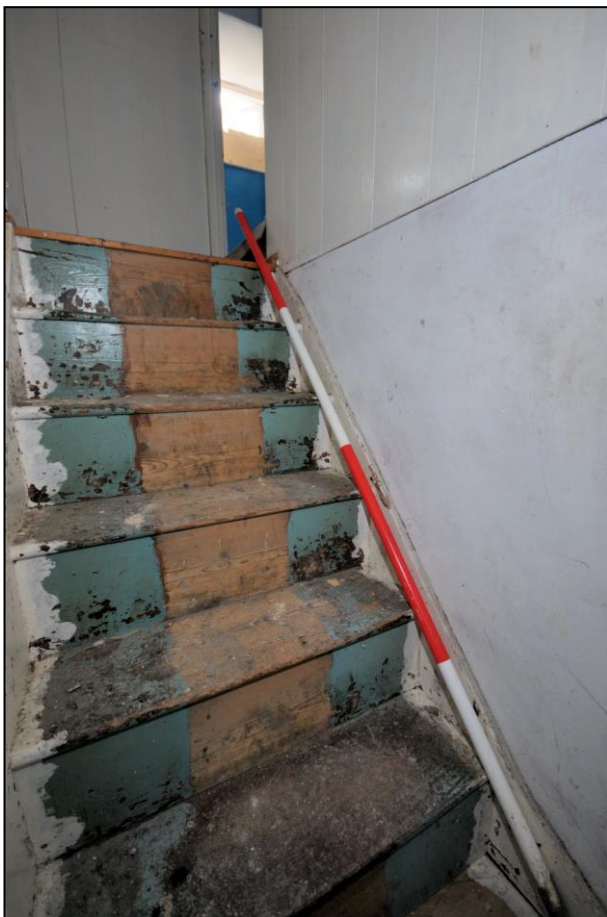
Image 22: No. 41, stairs, looking up Facing south-east (Scale 2m)
