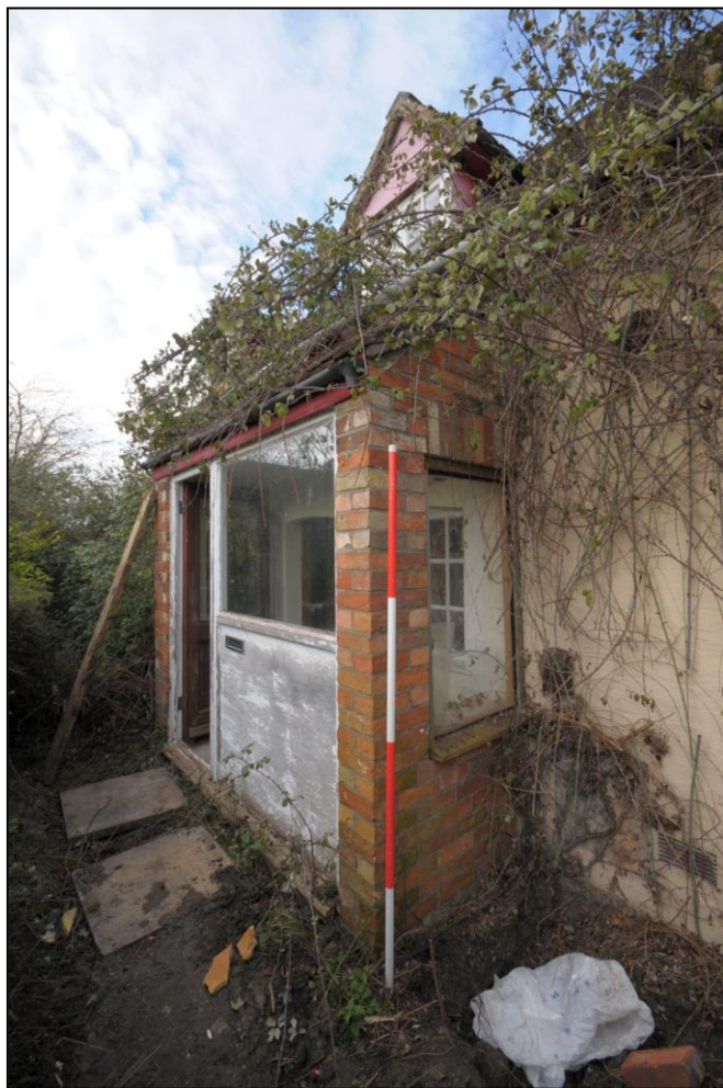
Image 5: South elevation, porch Porch of No. 41. (Scale 2m)
