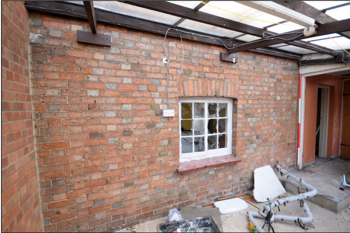
Image 17: No. 41, conservatory, looking south-east Rear wall of primary range (Scale 2m)
