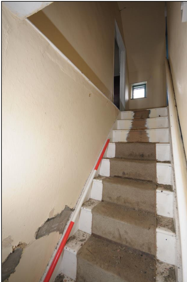
Image 40: No. 43, stairs, looking up
