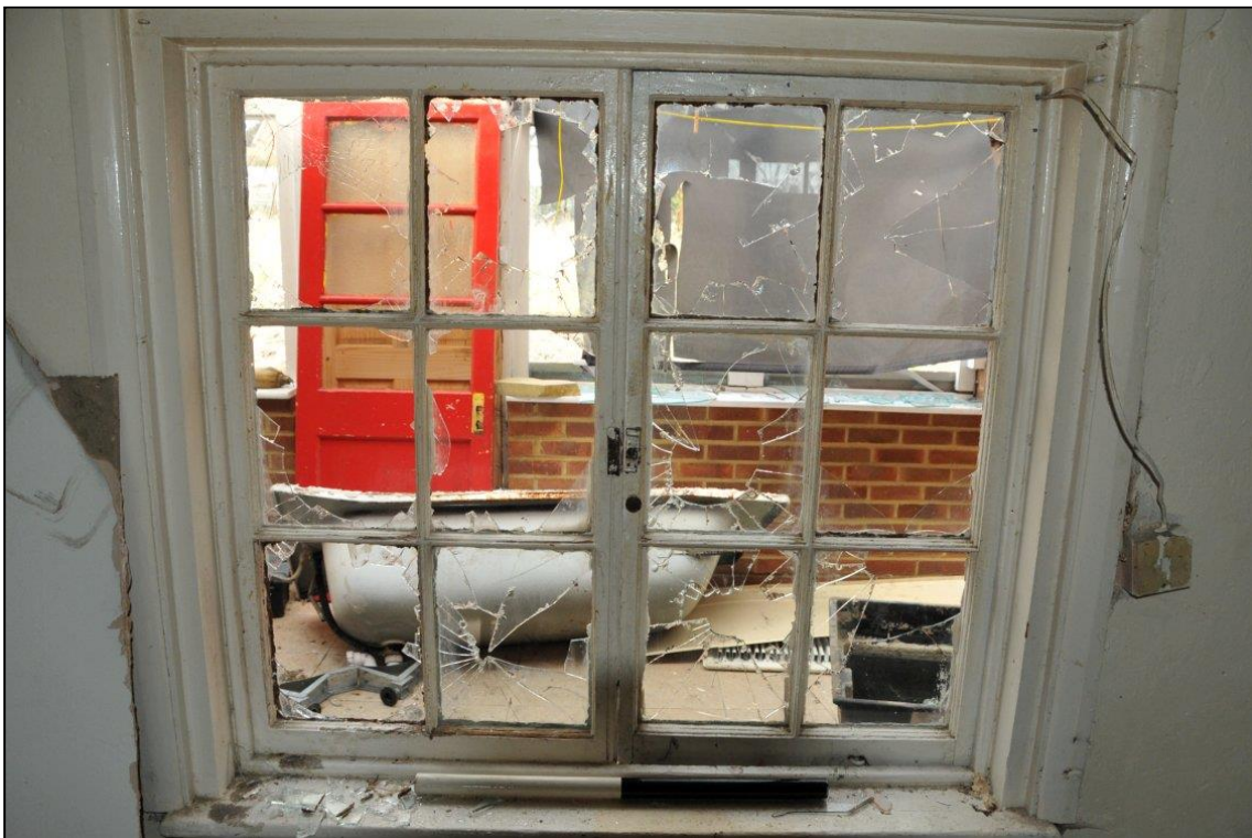
Image 12: No. 41, living room, detail of window in west wall
