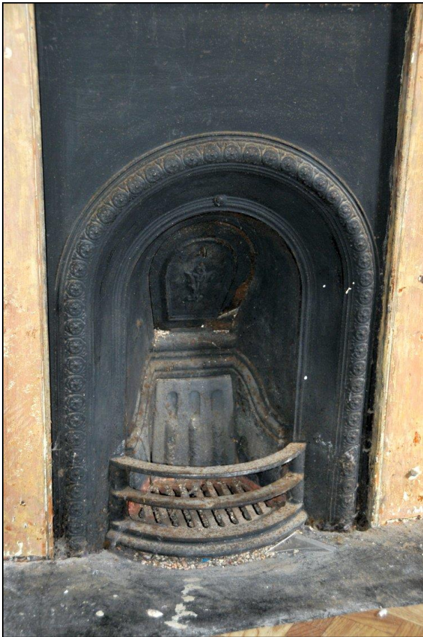
Image 27: No. 41, bedroom 1, detail of fireplace
