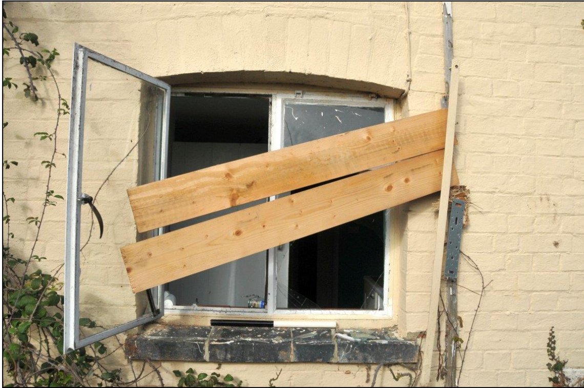
Image 3: South elevation, detail of window
