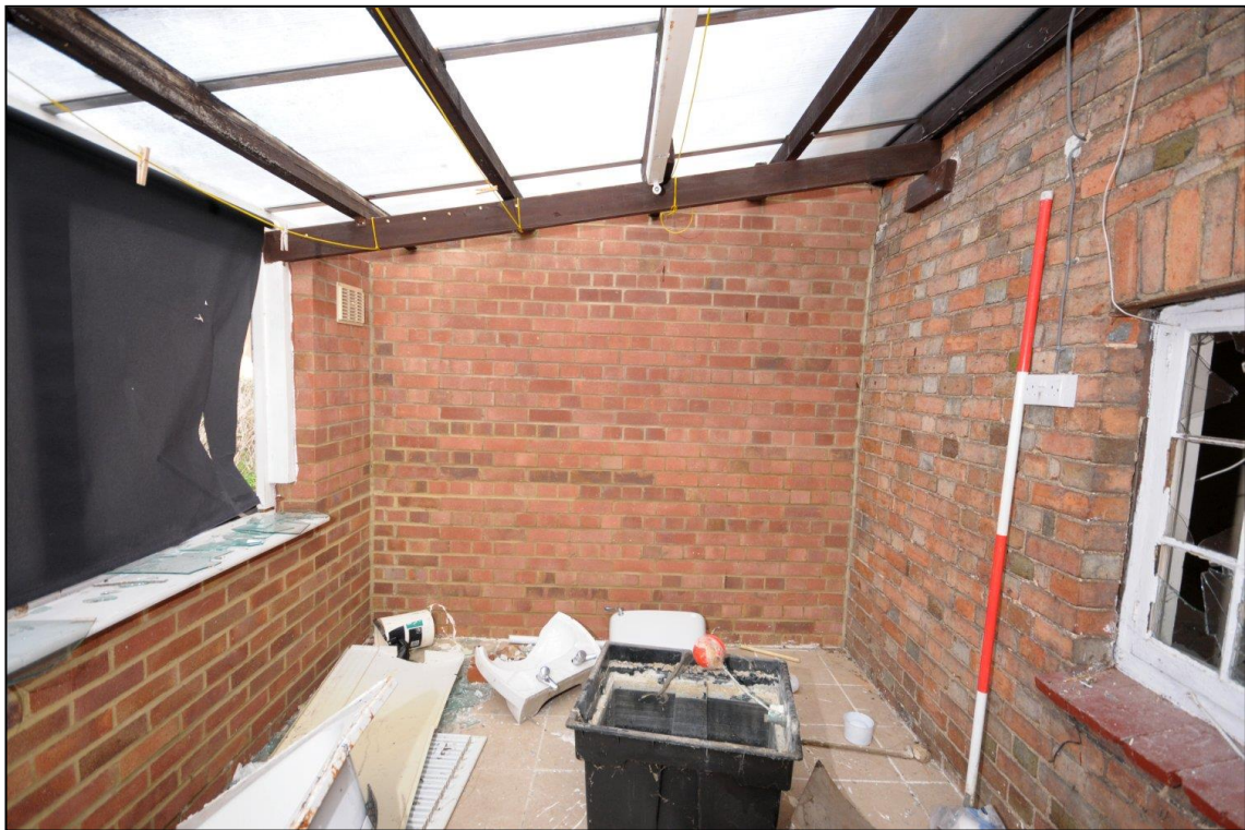
Image 20: No. 41, conservatory, looking north
