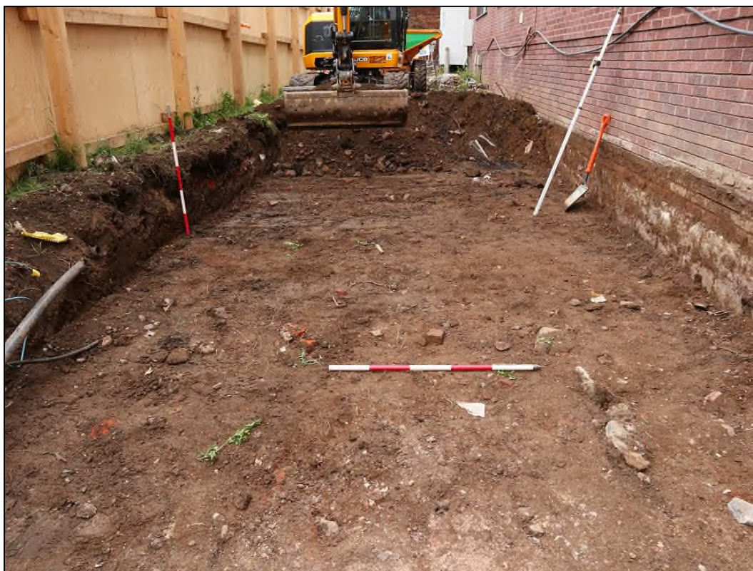
Image 1: Trench, looking east (Scale 2 x 1m)
