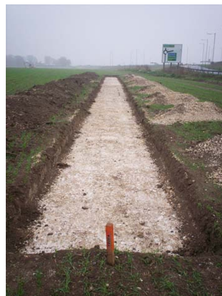
Trench 59: looking east-north-east. Scale 1m
