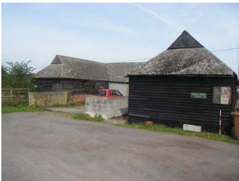
Figure 6: Warren Farm: outbuildings (view north)
