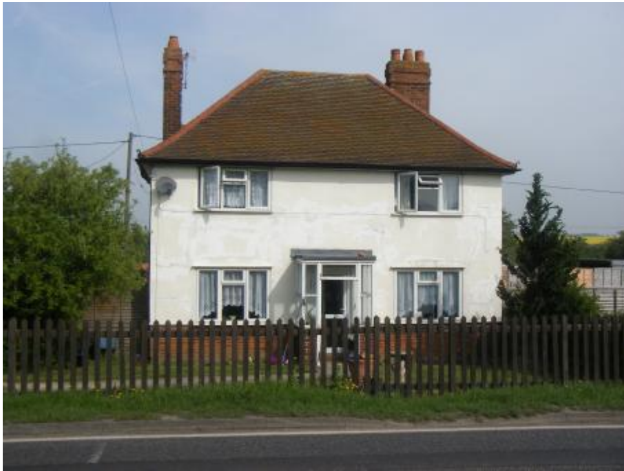
Figure 3: Warren Farmhouse: front (south) elevation
