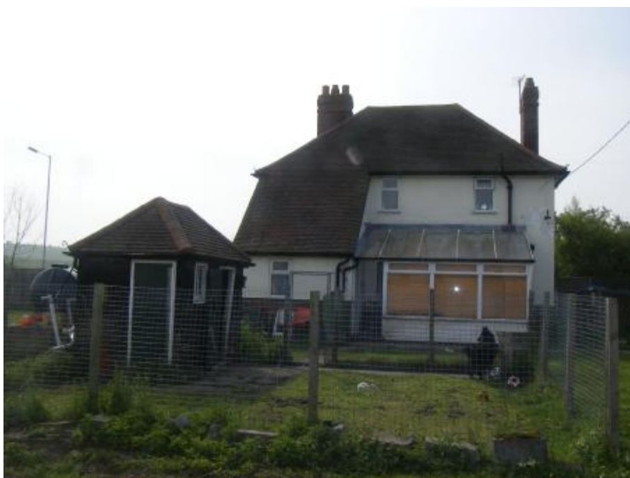
Figure 5: Warren Farmhouse: north elevation
