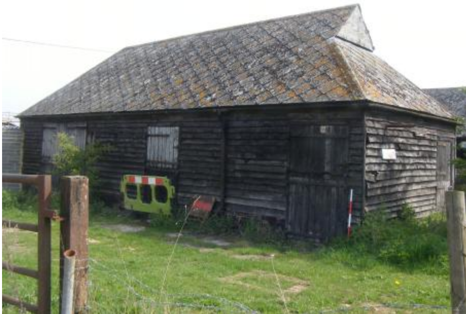
Figure 8: Warren Farm: outbuildings, western range (view north-east)
