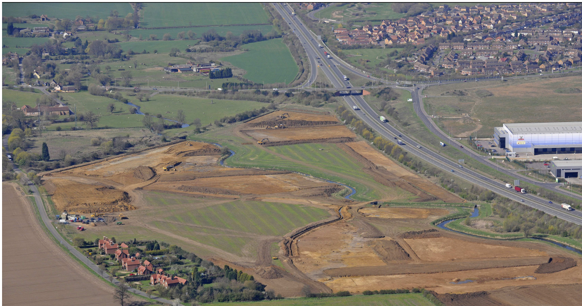
View from east of earthmoving halfway through the investigations
