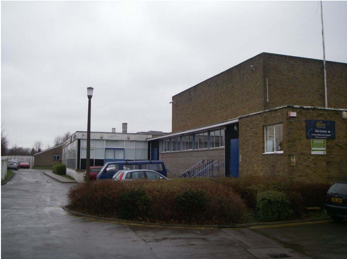
Figure 4: North-eastern elevation showing assembly hall and original 1947 brick and concrete clad classrooms. 1967 SEAC Mark 2 building to the left.
