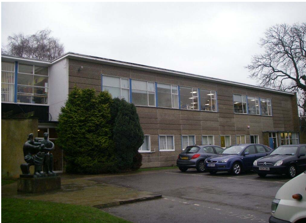
Figure 3: South-eastern elevation with Henry Moore sculpture in front of main entrance to the left. Note concrete cladding typical of the Hertfordshire 8'3" System
