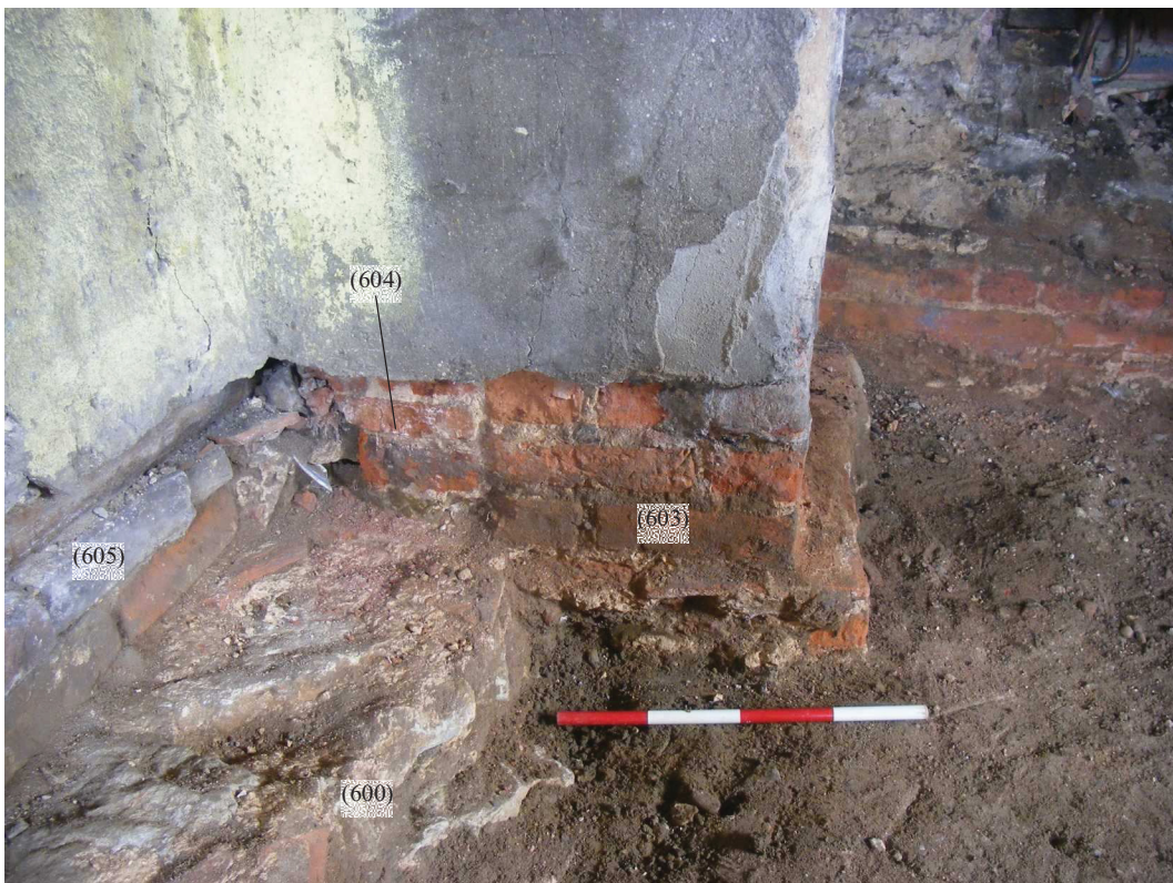
Photo 6: Brickwork infilling adjacent to the fireplace in the lobby-entry dwelling
