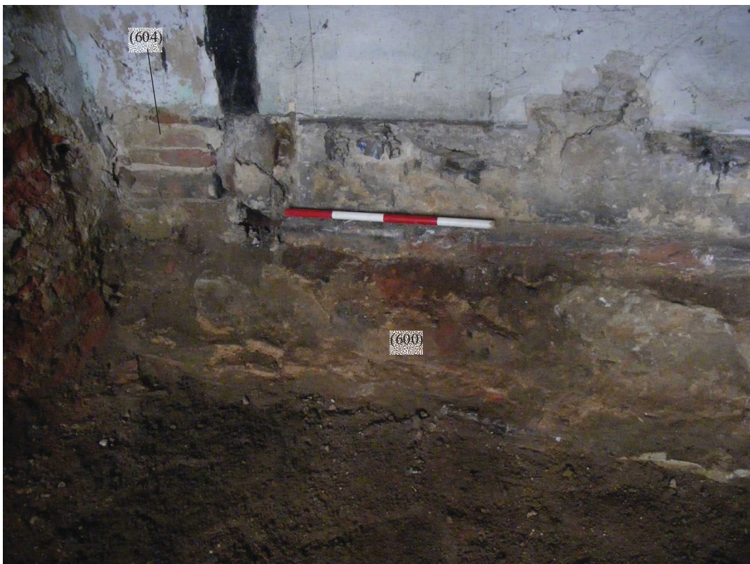
Photo 2: Brickwork in north corner of 'dining room'
