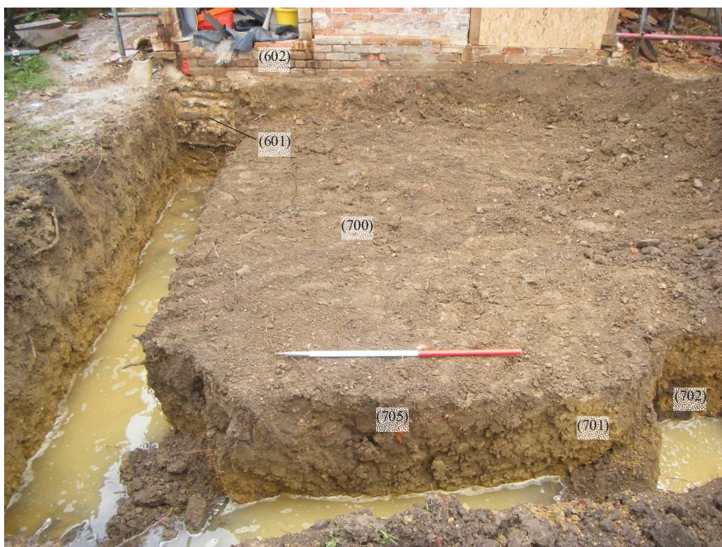
Photo 17: Features observed in the foundation trench for the new build extension
