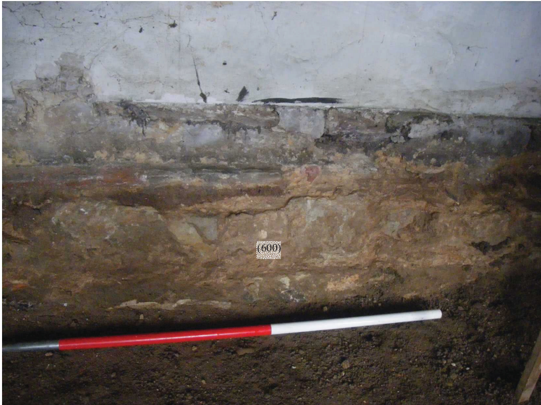
Photo 1: Foundations in the 'dining room' of the lobby-entry dwelling
