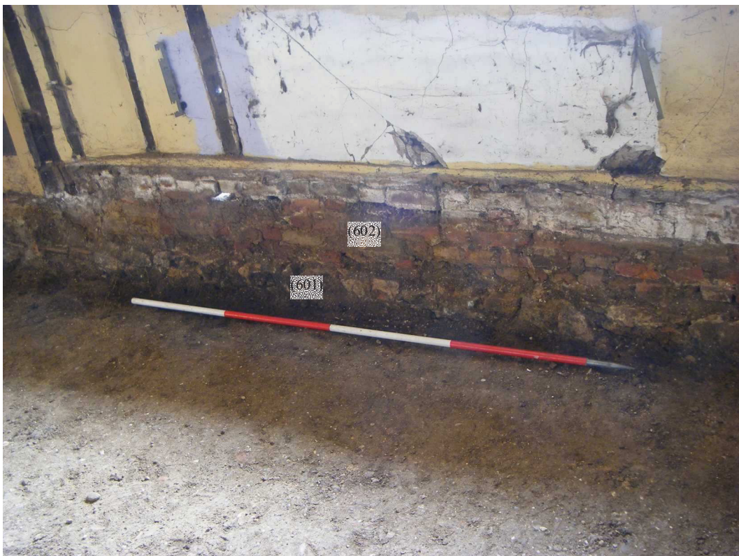
Photo 12: Foundations, dwarf wall within the end-stack dwelling
