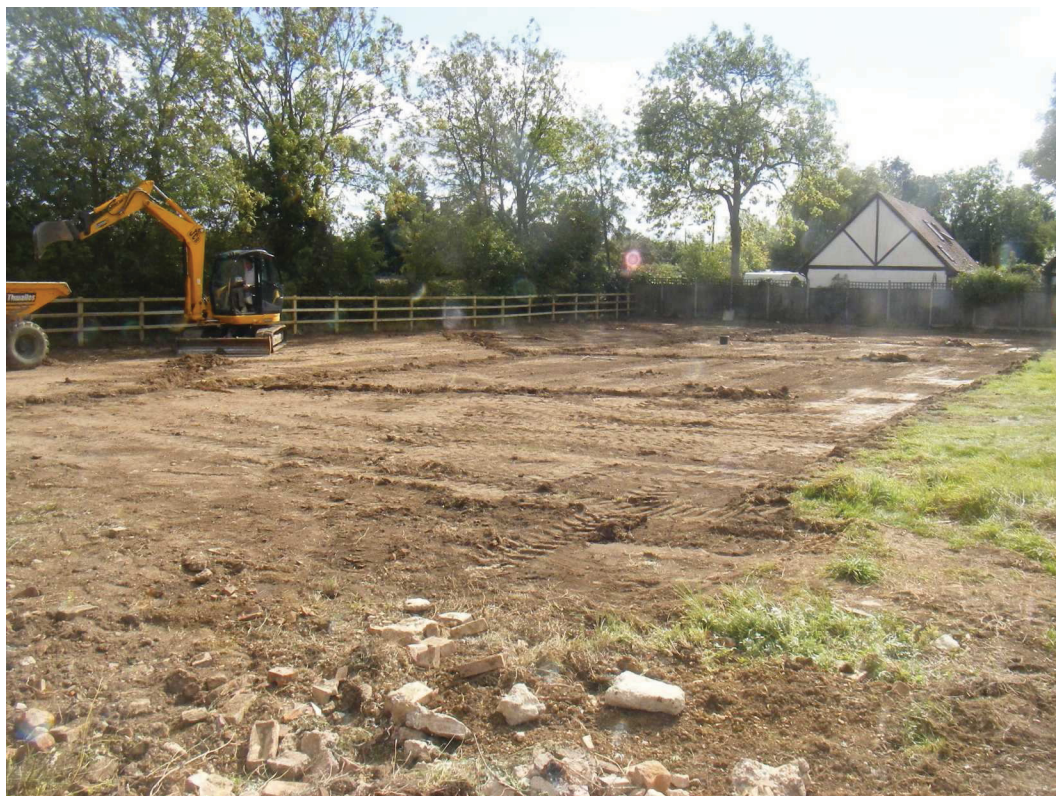
Photo 19: The manège under construction.
