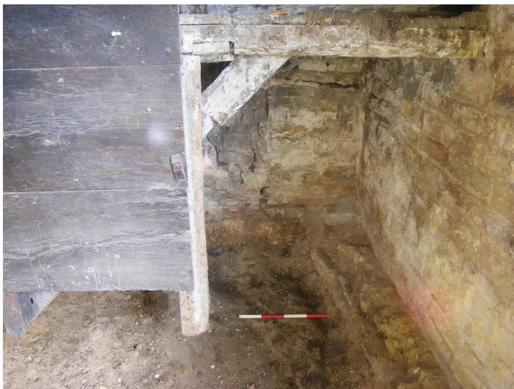
Photo 3: Foundations of north-west gable of lobby-entry dwelling
