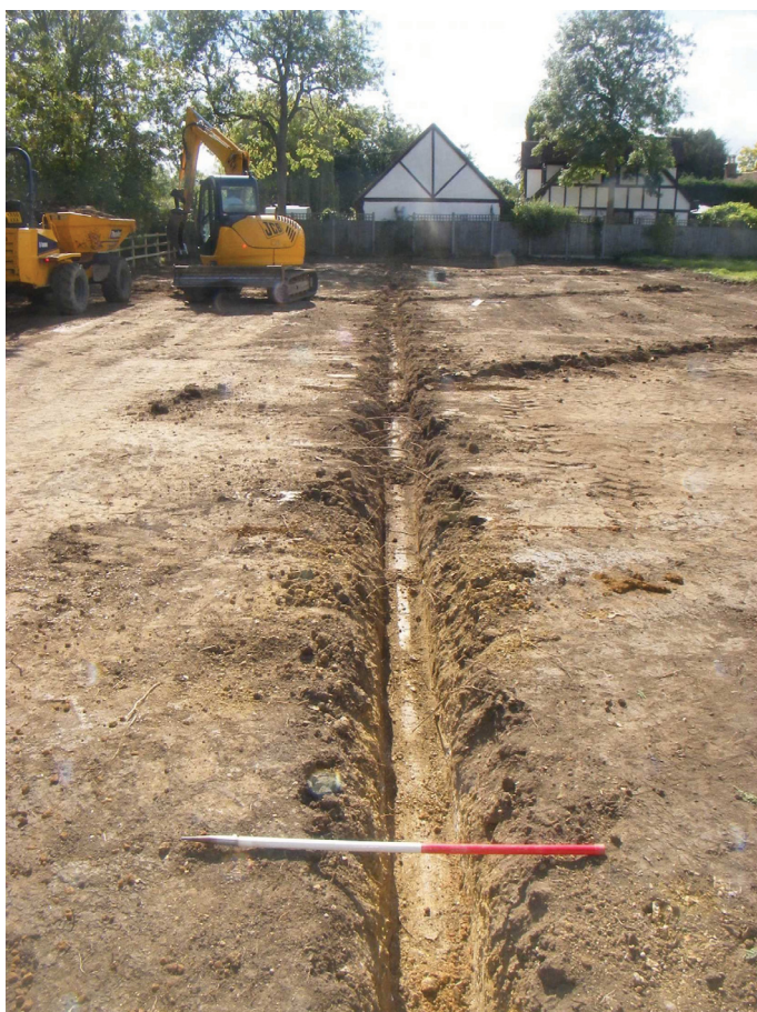
Photo 20: The manège, showing main axial land-drain trench.
