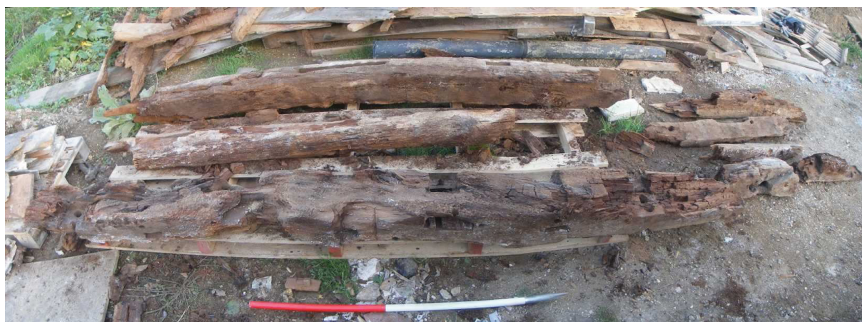
Photo 8: Former structural timbers re-used as sleepers beneath the floor boards in the end-stack dwelling
