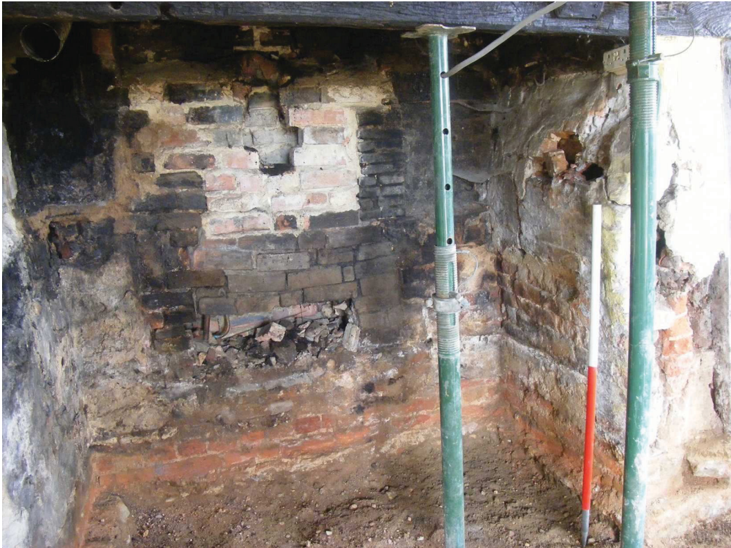
Photo 9: Brickwork at the back of the 'kitchen' fireplace
