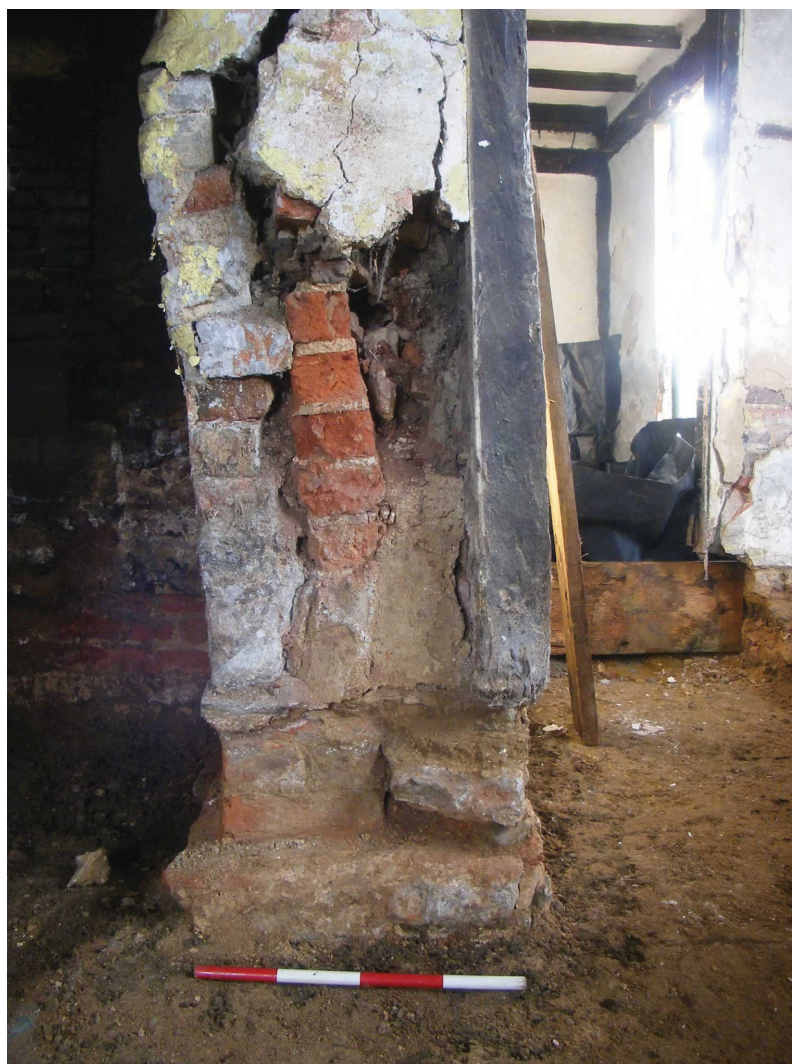
Photo 7: Detail of construction, right-hand pier of the fireplace
