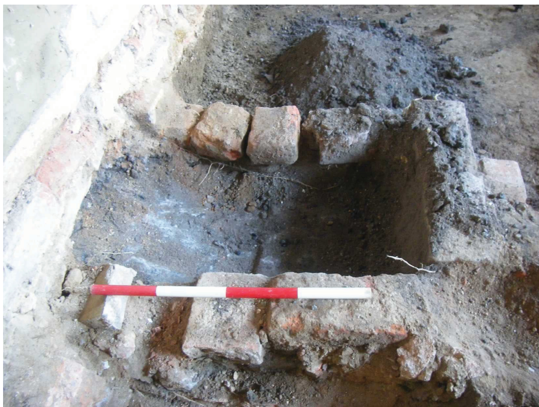
Photo 16: 'Ash chute' collection box (608) with fill removed (Note the bricked-up void beneath the timber sill.)
