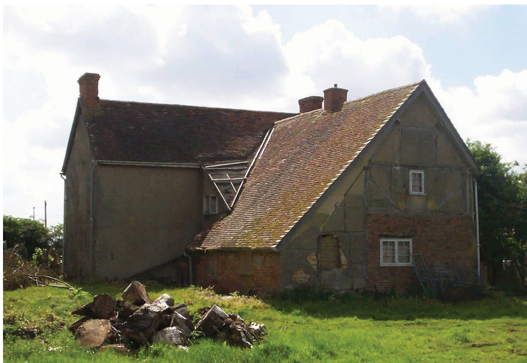
Photo 4: North-west gable of lobby-entry dwelling, exterior view
