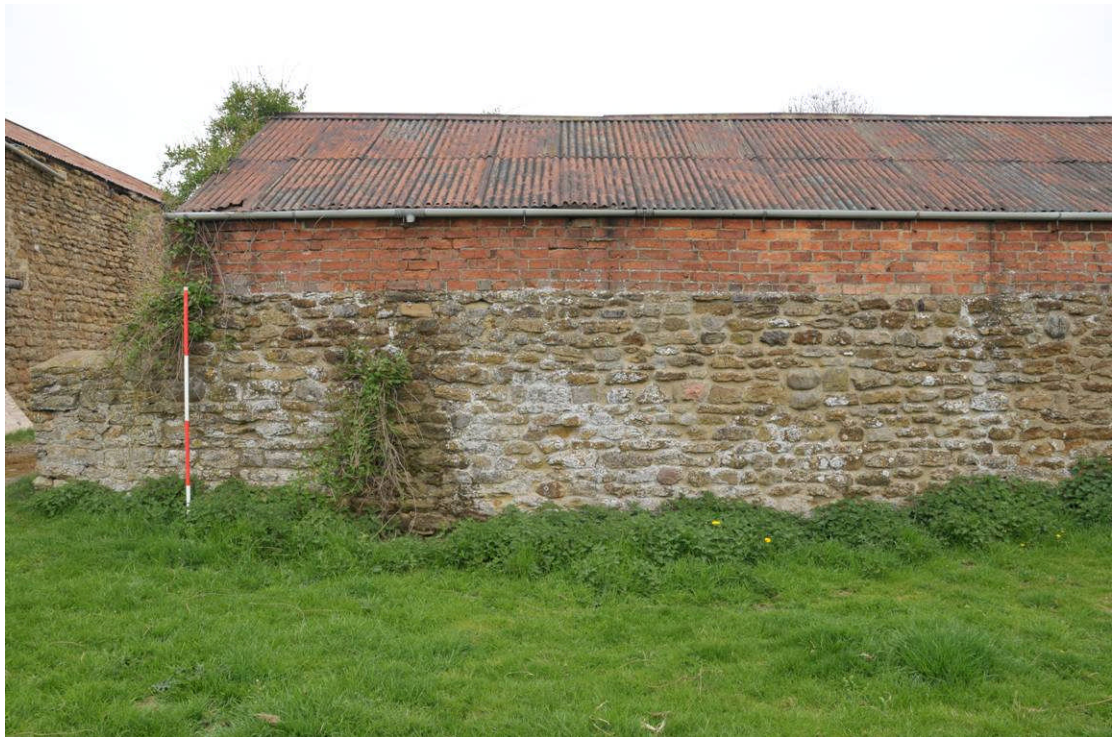
Plate 28: Open-fronted shed (Building E), western elevation
