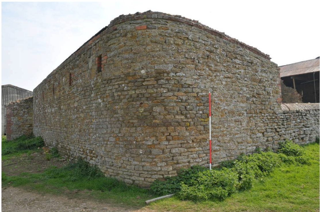
Plate 23: Open-fronted shed (Building D), western and northern elevations
