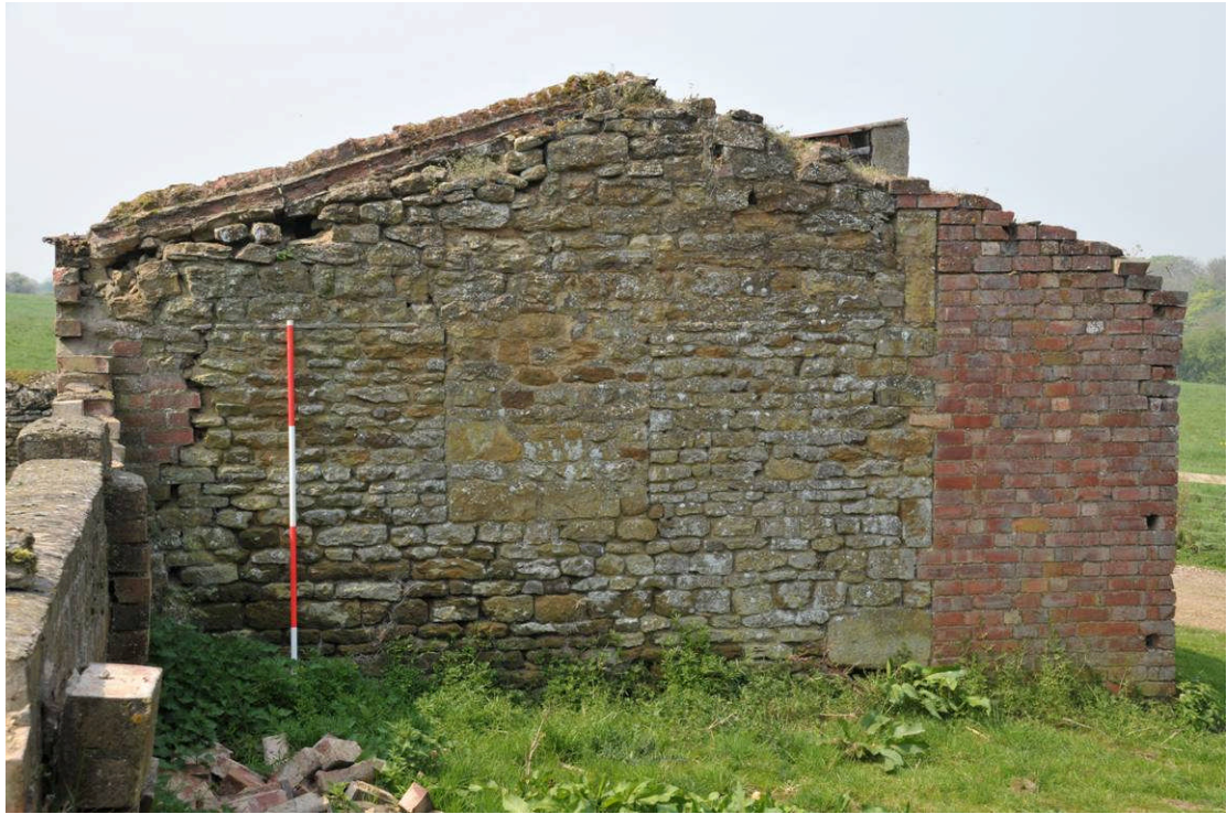
Plate 24: Open-fronted shed (Building D), eastern elevation
