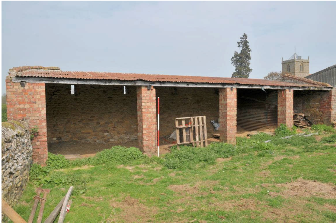
Plate 22: Open-fronted shed (Building D), southern elevation
