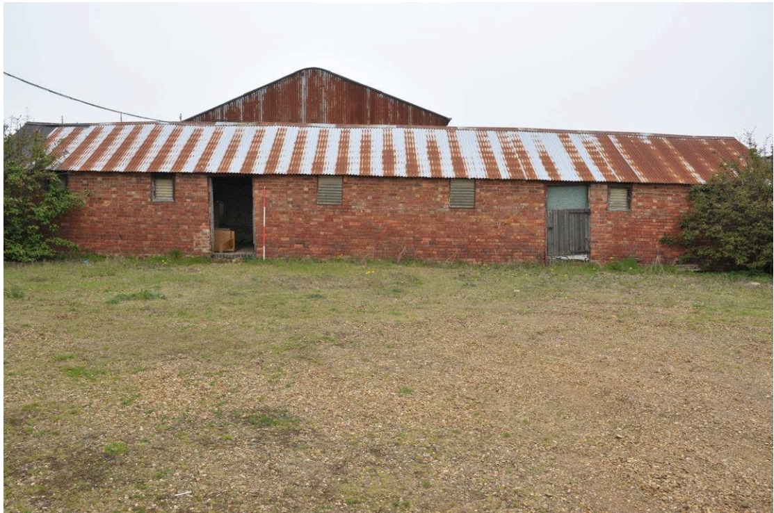
Plate 4: Cow house (Building B), Private Courtyard
