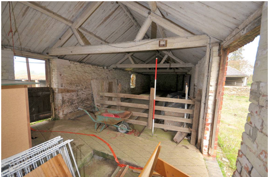
Plate 11: Cow house (Building B), interior
