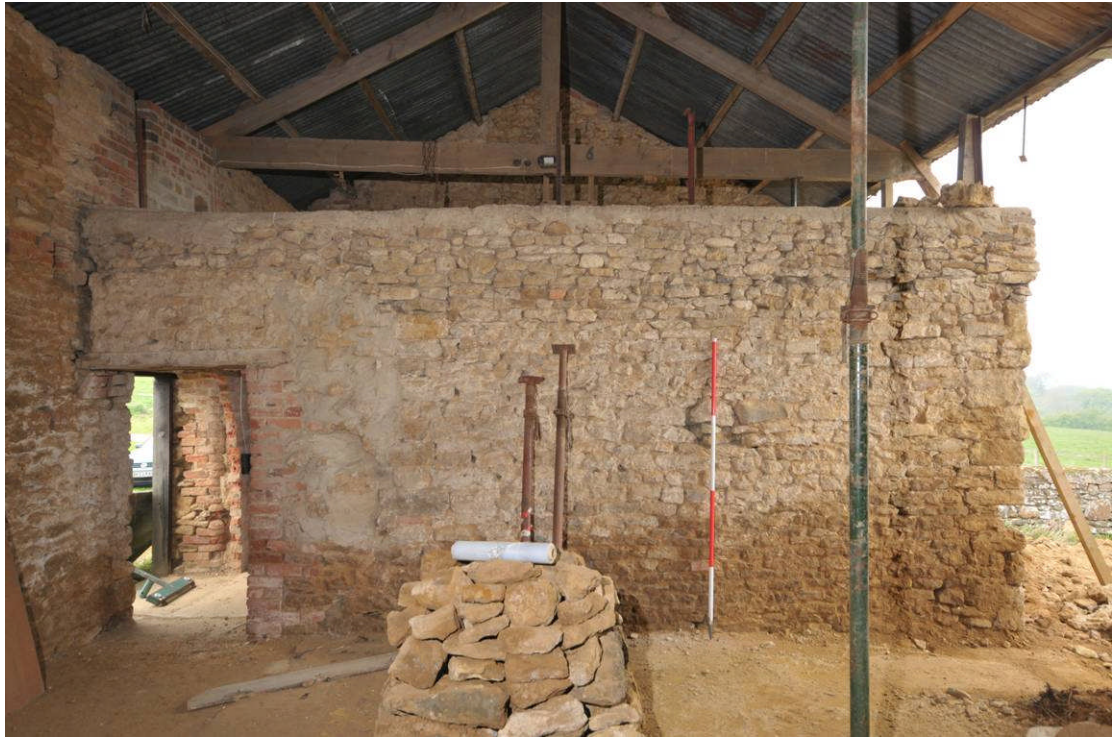
Plate 20: Barn (Building C), interior, partition wall
