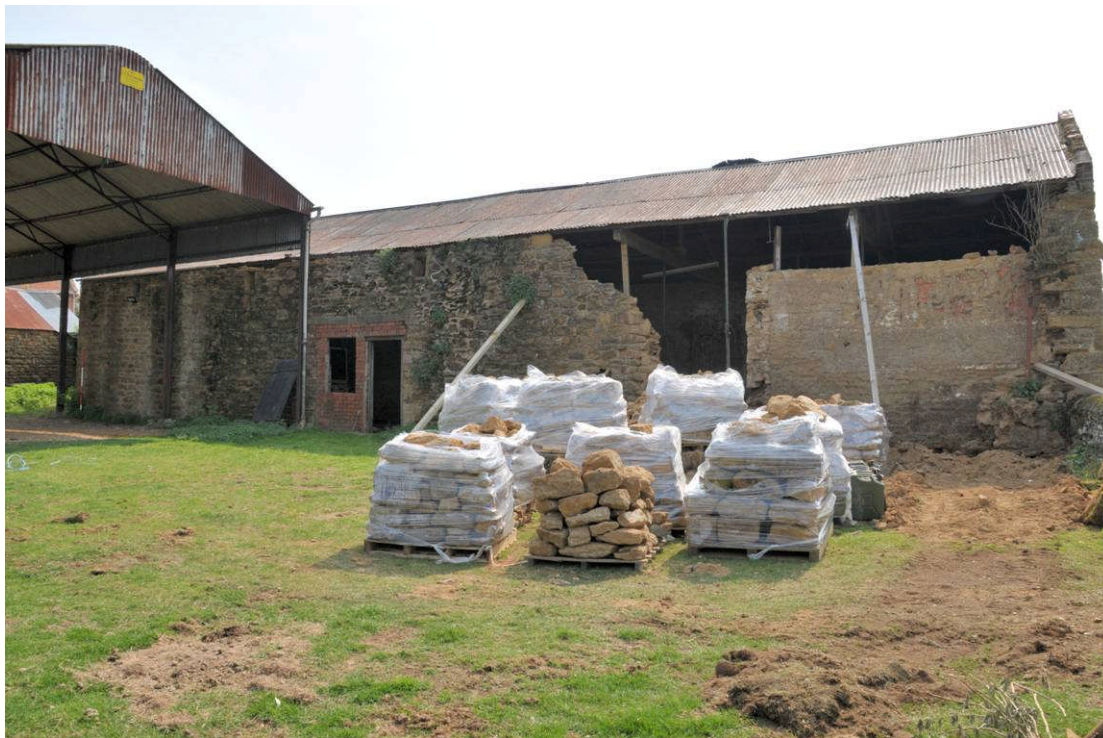
Plate 13: Barn (Building C), northern elevation
