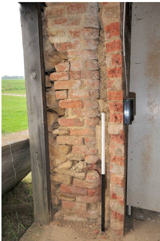
Plate 21: Barn (Building C), detail of door opening, west end
