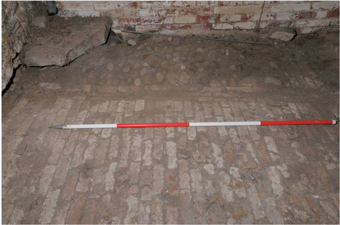
Plate 10: Cow house (Building B), detail of floor
