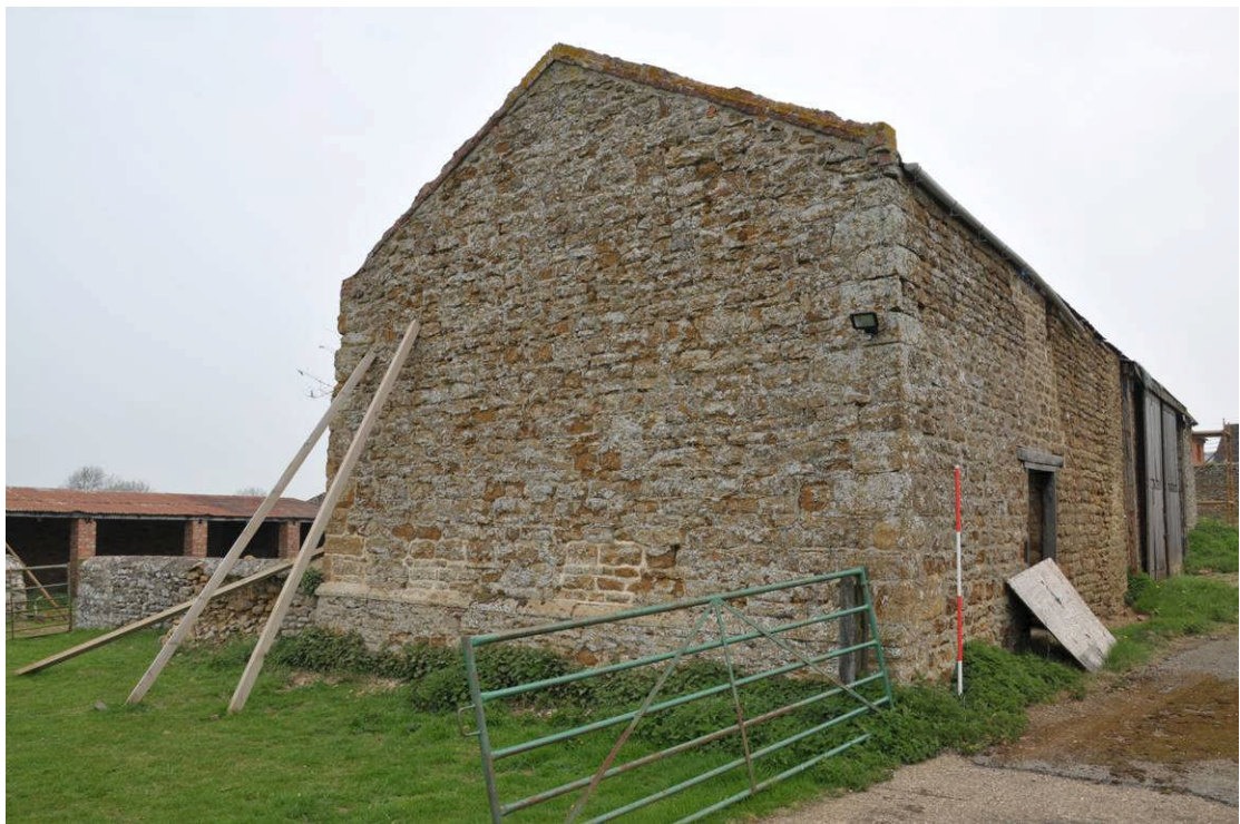
Plate 15: Barn (Building C), western elevation
