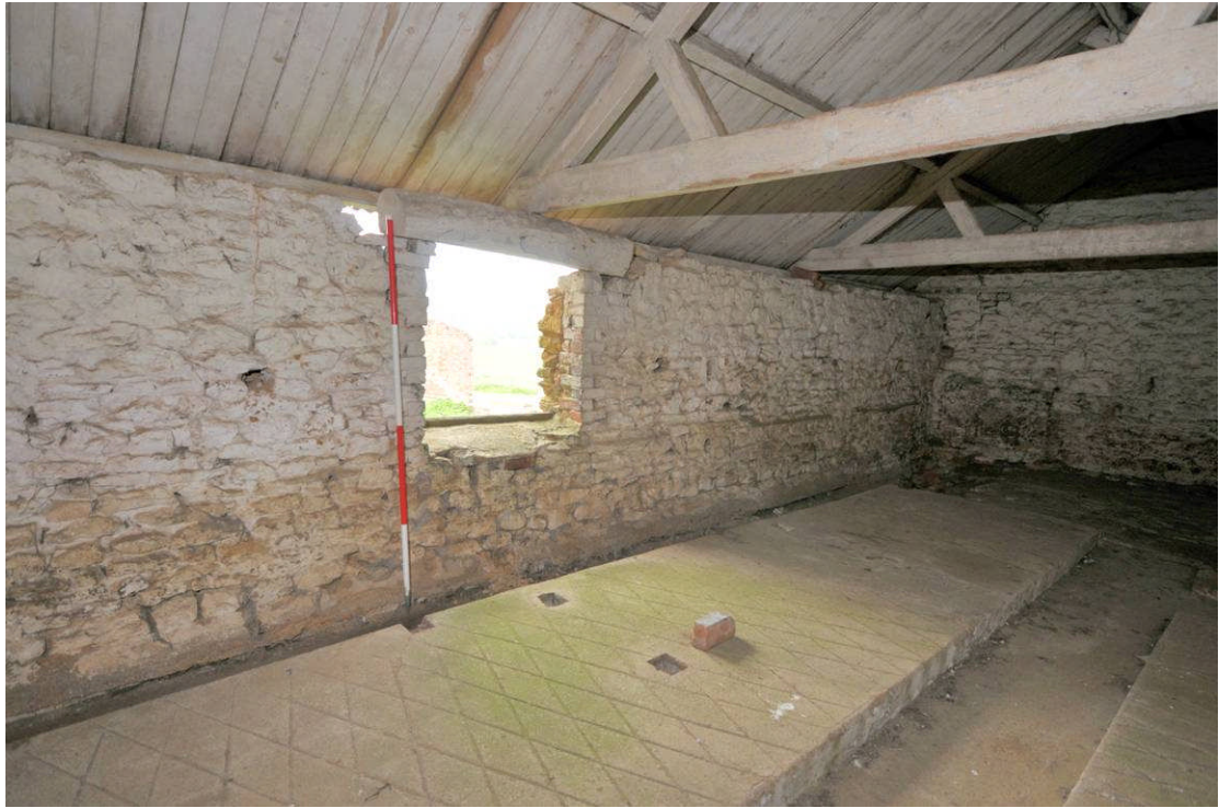
Plate 8: Cow house (Building B), interior
