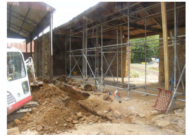
Photograph of the threshing barn trenches. Looking east.
