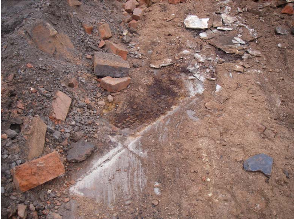
Figure 18: Trench 4, asbestos plates above concrete slab
