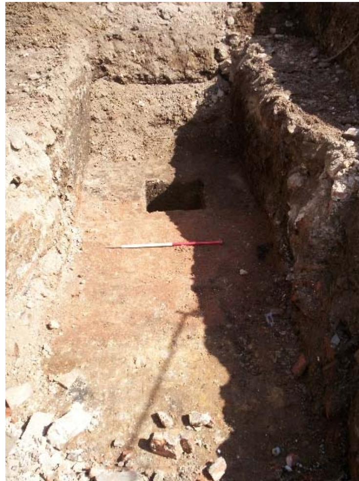
Trench 2 looking east (1m scale)
