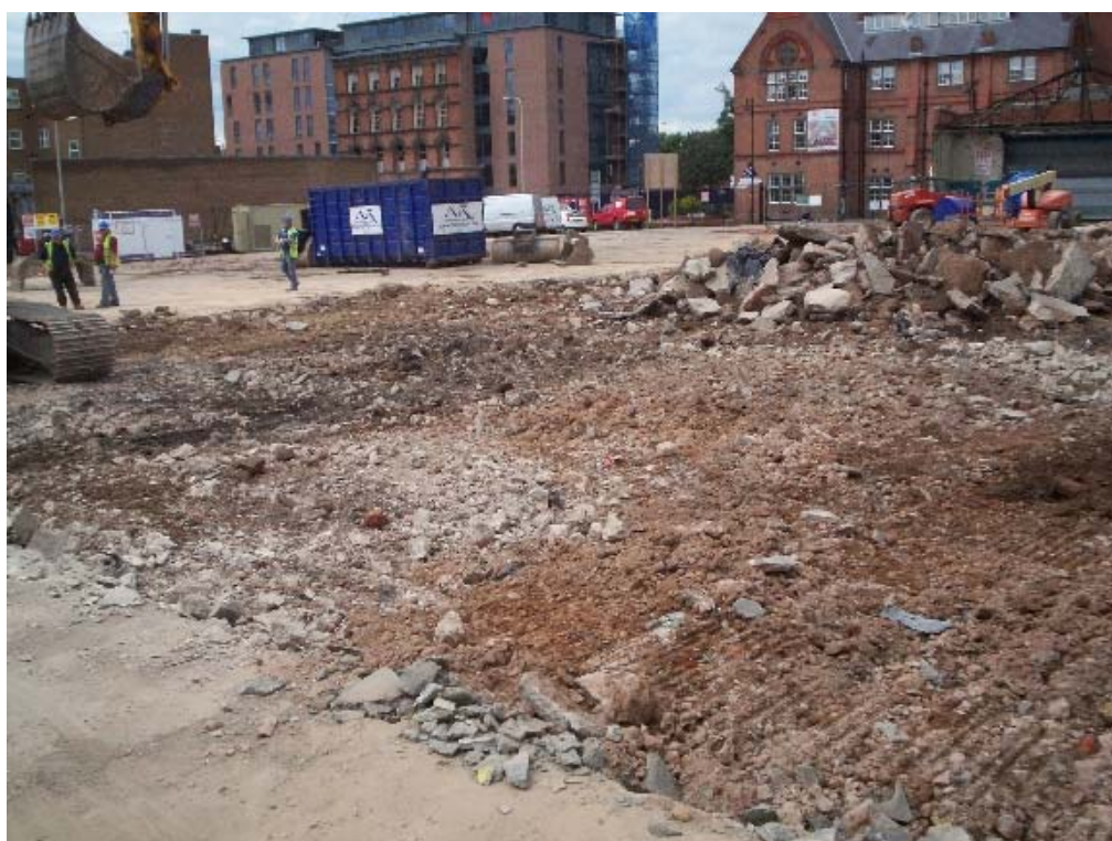
Figure 13: Rubble layers exposed after removal of concrete slab
