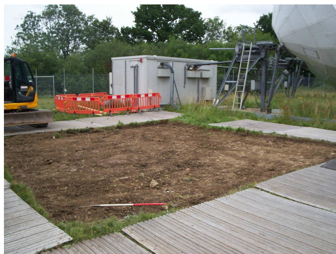
Photograph of trench immediately after turf removal. Scale 1m. Looking north-east.
