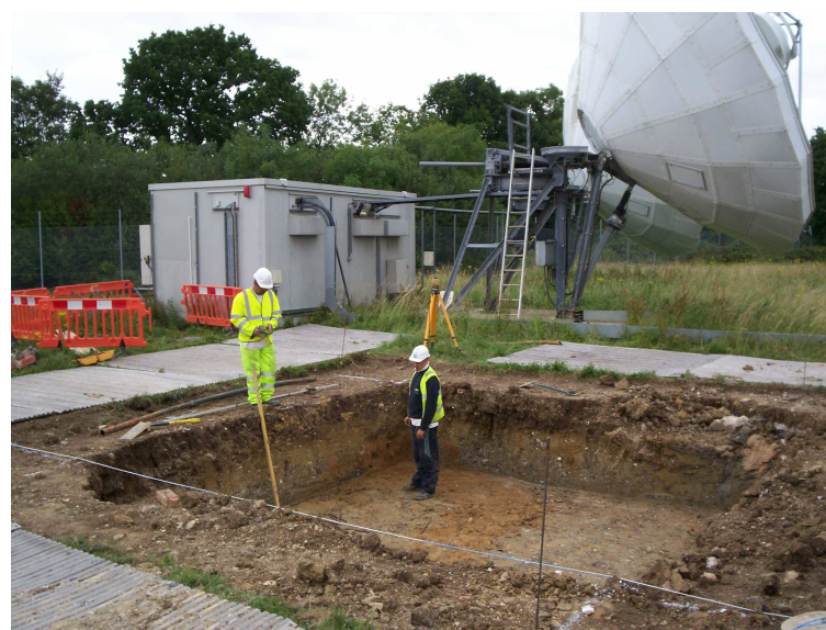
Photograph of trench showing full excavated depth. Looking north-east.
