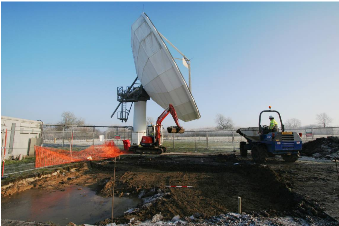
Image B: General view of trench (looking east)
