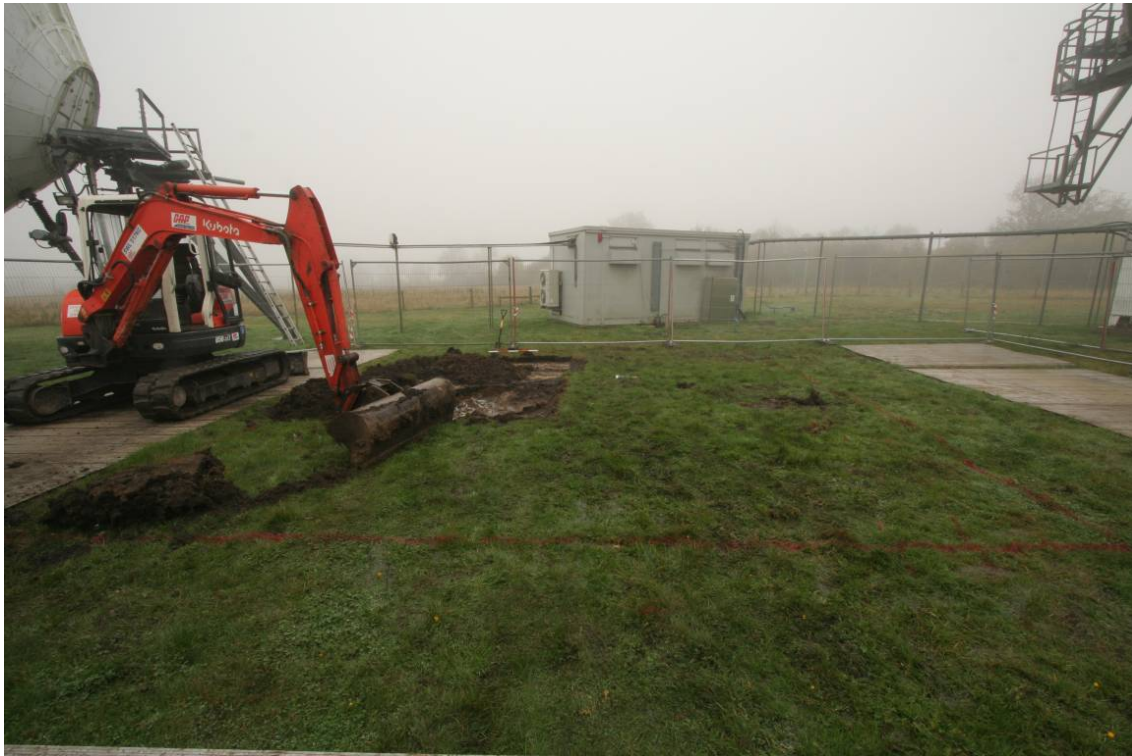
Image A: Showing site at start of ground works (looking north)
