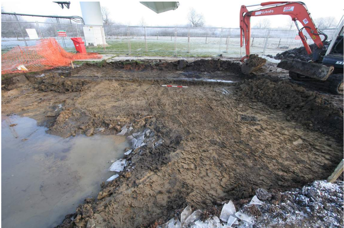
Image D: View of trench looking east
