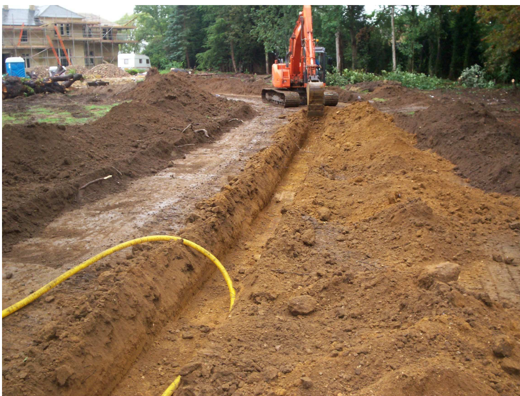
Image 2: Cutting drainage trench along driveway, exposing the undisturbed geological strata.
