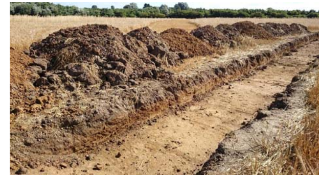
Trench 89 compacted soil at west end
