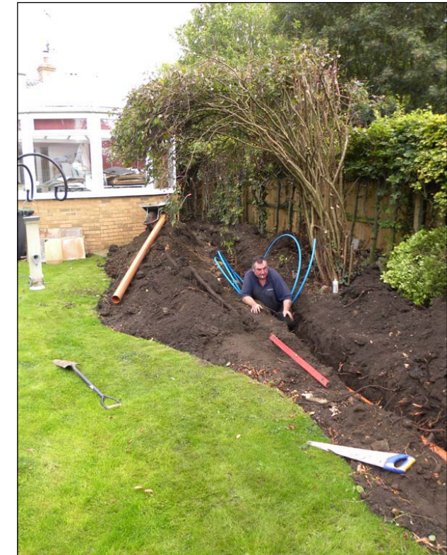
Photograph 1: general view of drainage trench from western end
