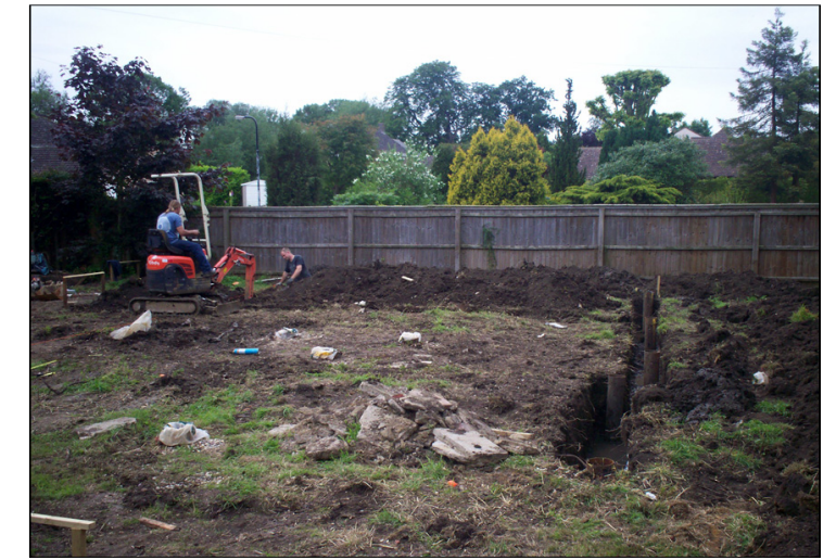
Photograph 3: general view of house footings, looking west
