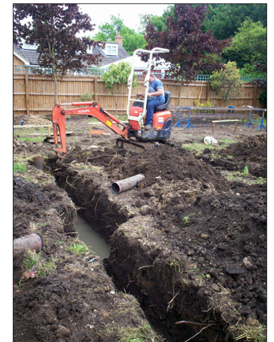
Photograph 4: general view of house footings, looking east
