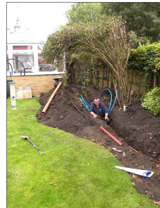
Photograph 2: general view of drainage trench, looking east
