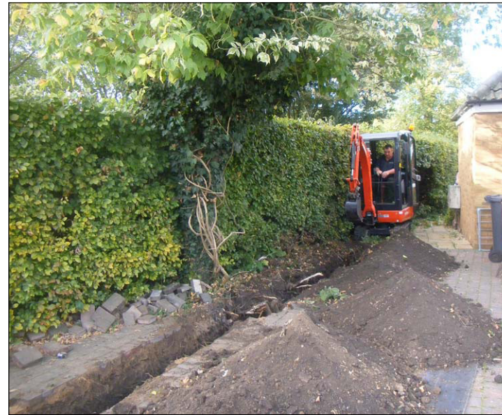
Photograph 1: general view of drainage trench, looking west
