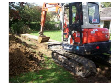
Machining of trench
