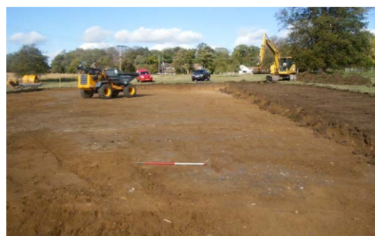
Photograph 1: Machining of manège, looking north
