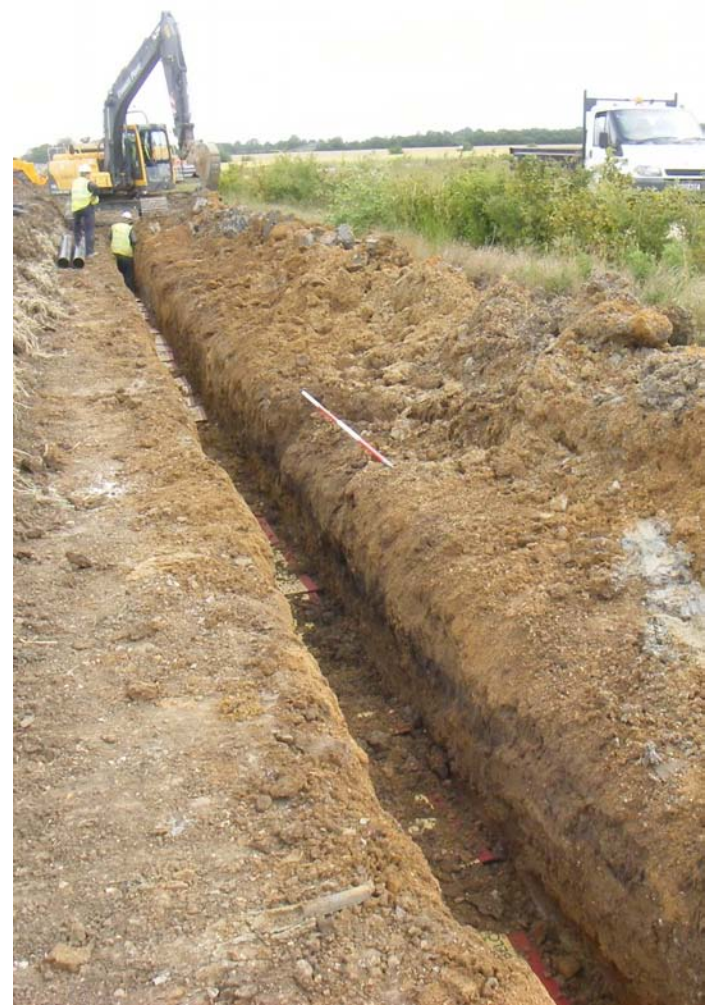
Photograph of ditch [2106]. Looking north east. Scale 2m
