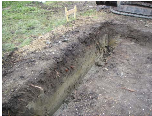
North edge of foundation trench. Looking E.
