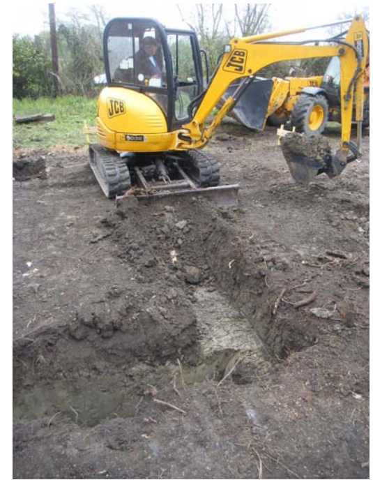
Excavation of trench. Looking NE
