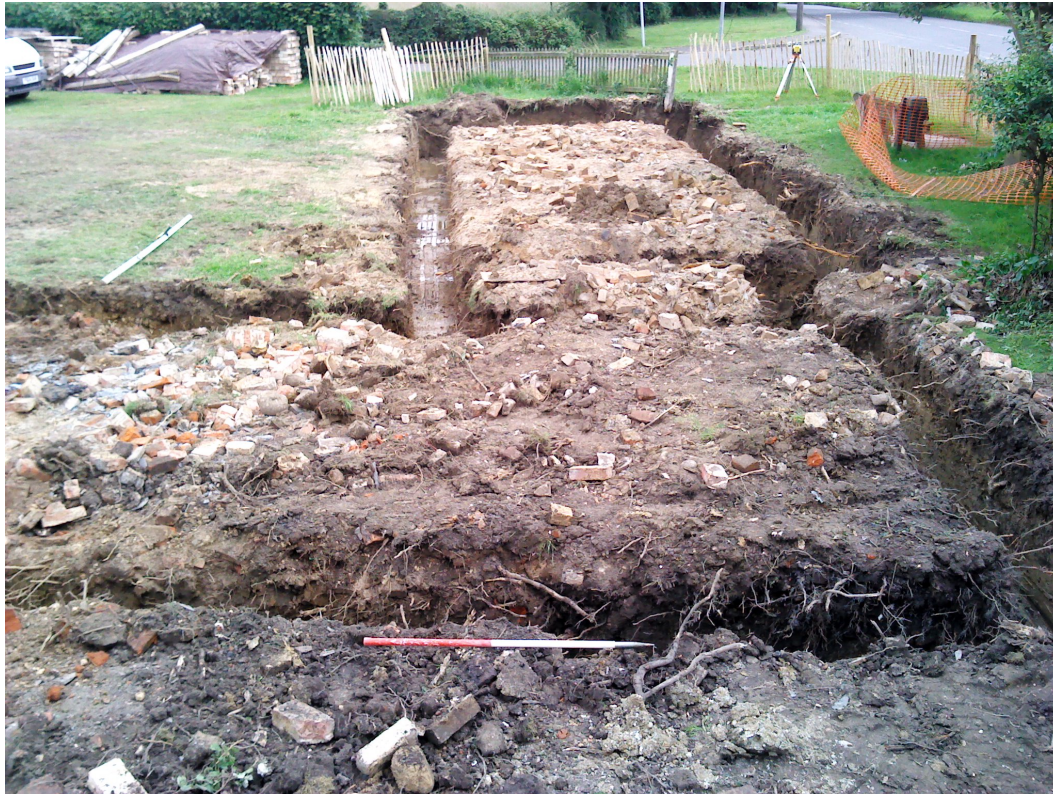
Figure 21: General view of excavated footings
