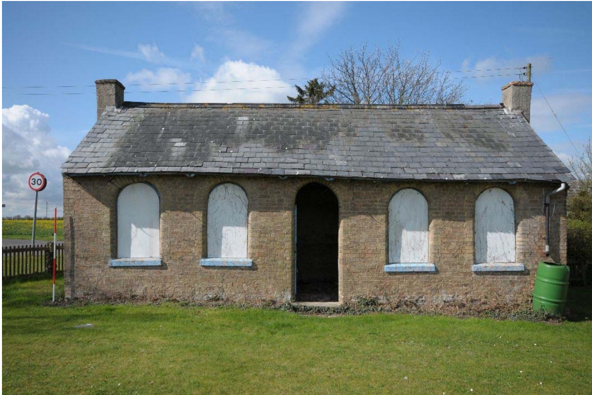
Figure 12: School room, east-facing side
