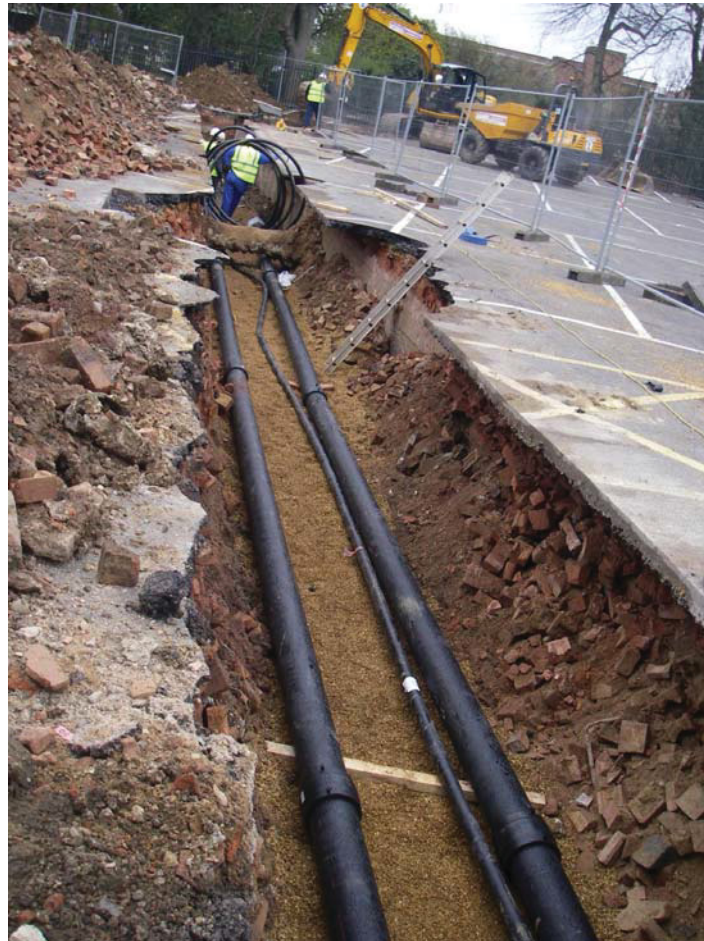
Image 1: Trench through Bedford College car park Looking north
