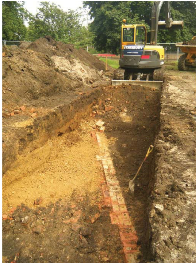
Image 4: Brick foundations in St Mary's Gardens
