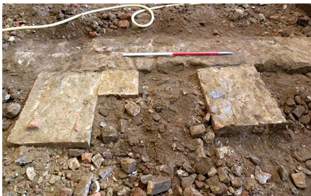
Image 4: Eastern face of ironstone wall with later plinths butting-up. Scale 1m in 50cm divisions.
