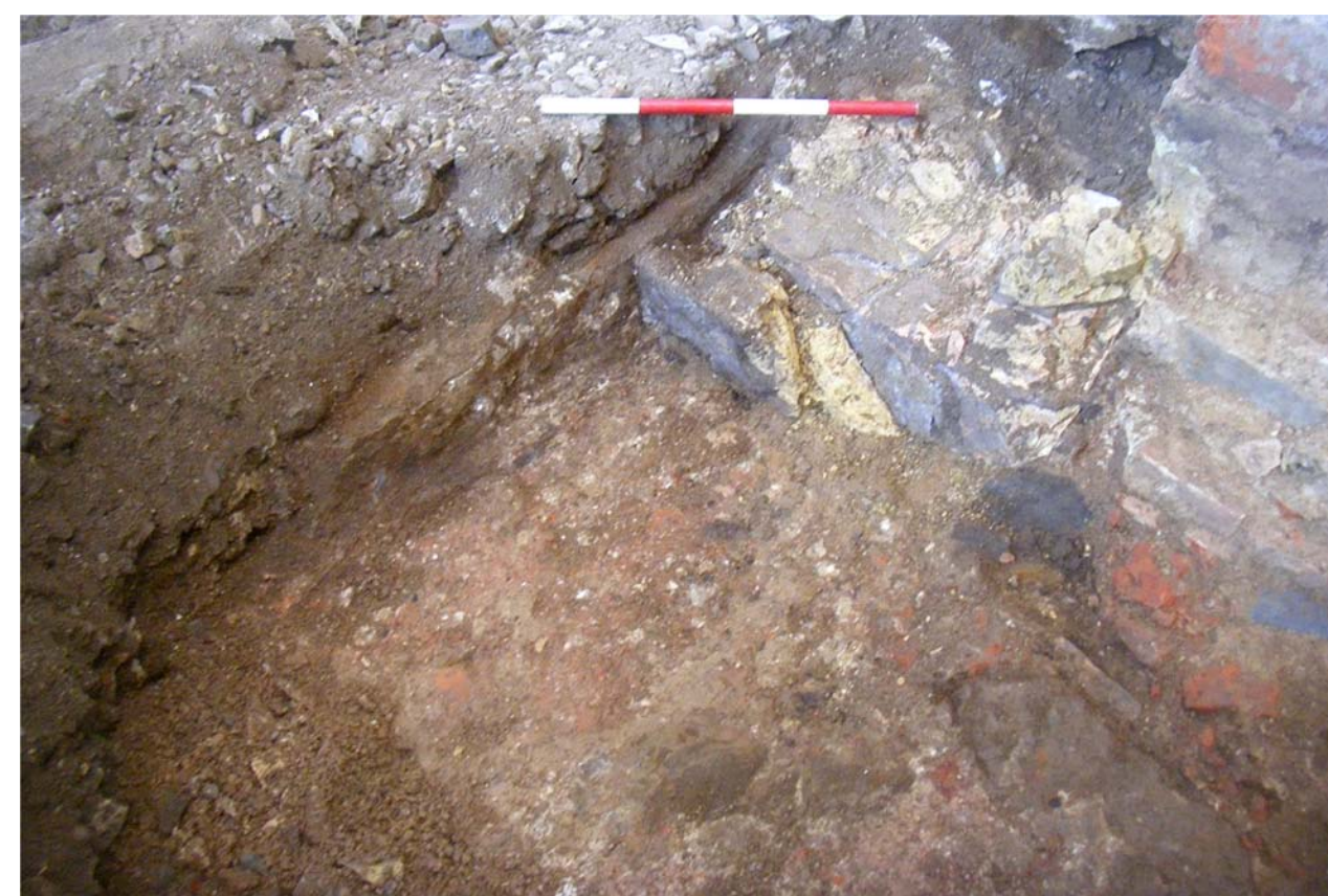
Image 6: The interior (western face) of the eastern gable of the Ironstone mill is just visible extending from the section. Beyond the buttress are the damaged remains of a Fletton brick plinth base, with the partially robbed out footing of an Ironstone wall in the foreground — this is possibly an earlier phase of Ironstone mill. Scale 40cm in 10cm divisions.
