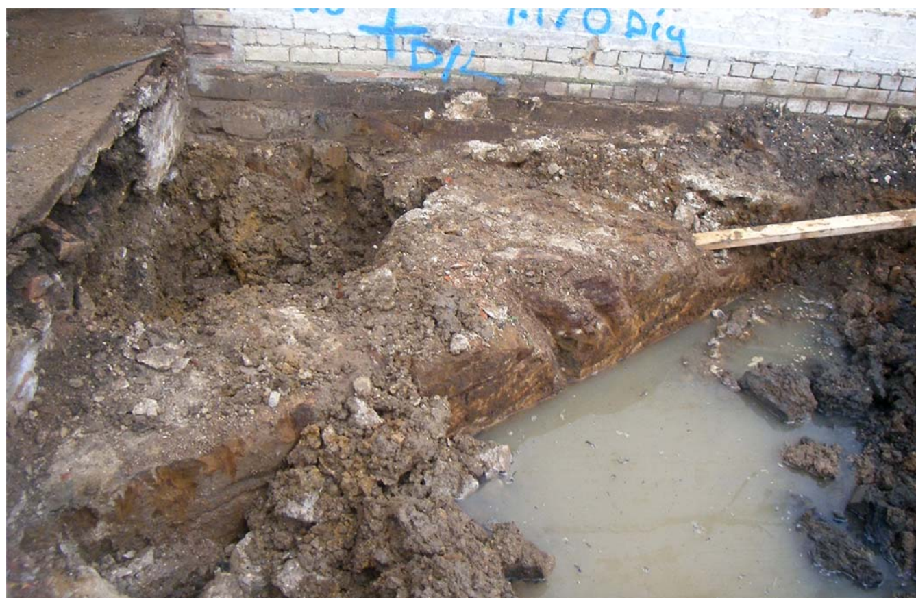
Image 8: General view of substantial Ironstone wall of the bypass leat, extending into southern elevation of the mill. Part of the Ironstone mill footing can be seen to the top left of the image — see image 10 below. Image 9: Detail of the intersection of the Ironstone wall and the mill. The red bricks appear to define a blocking of the channel, prior to the current mill (white bricks). Scale 25cm in 5cm divisions.
