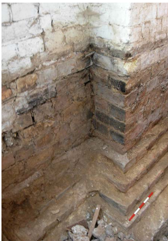
Image 1: Detail of stepped eastern gable wall of Mill Building revealed in the test pit, with Fletton bricks forming the superstructure — grey scar of modern concrete floor visible at top of image. Concrete underpinning is visible at the bottom of the image. Scale 25cm in 5cm divisions.
