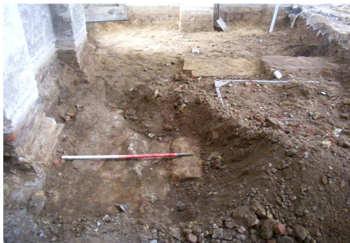
Image 5: Complex structural remains revealed beneath the modern mill floor. Evidence for possibly two phases of Ironstone wall footings was revealed. The earlier is visible underneath the photo scale — partly obscured by the stub of a later red brick E-W cross-wall, extending to the off-set buttress. Ironstone footings are visible beneath the brick walls of the standing mill, with the Ironstone eastern gable wall just visible at the limit of stripping — see image 6. Scale 1m in 50cm divisions.
