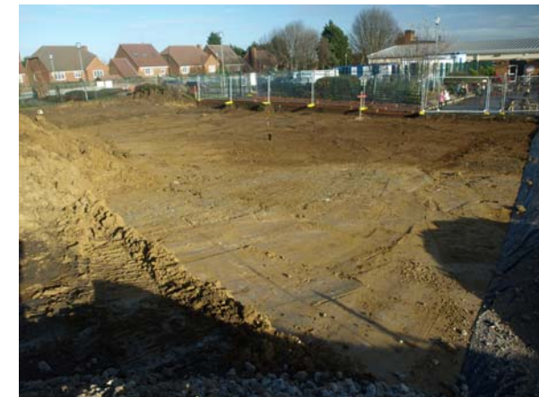
Post-ground reduction shot looking NE
