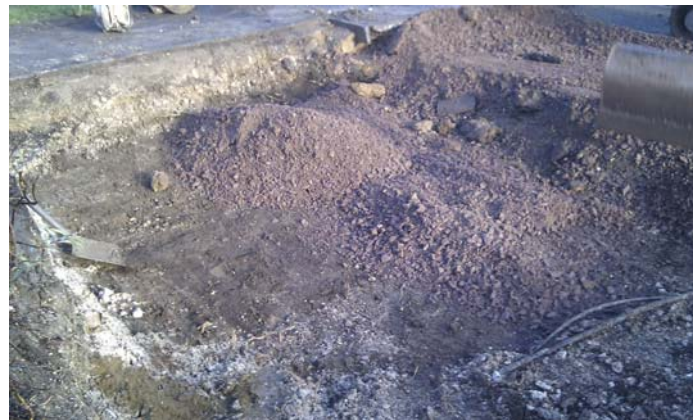
Western car park extension
