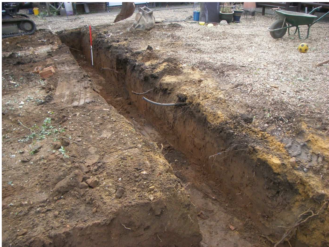
Figure 5: Southern foundation trench of new garage
