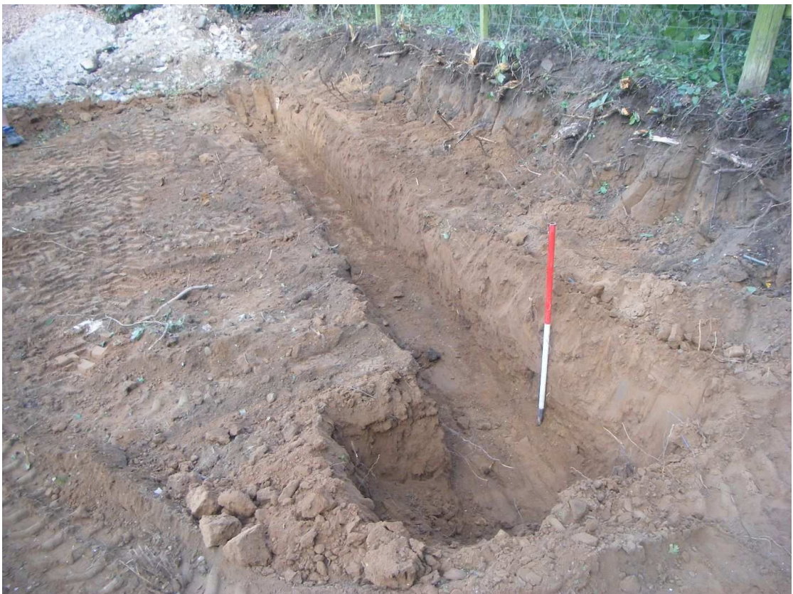
Figure 4: Northern foundation trench of new garage
