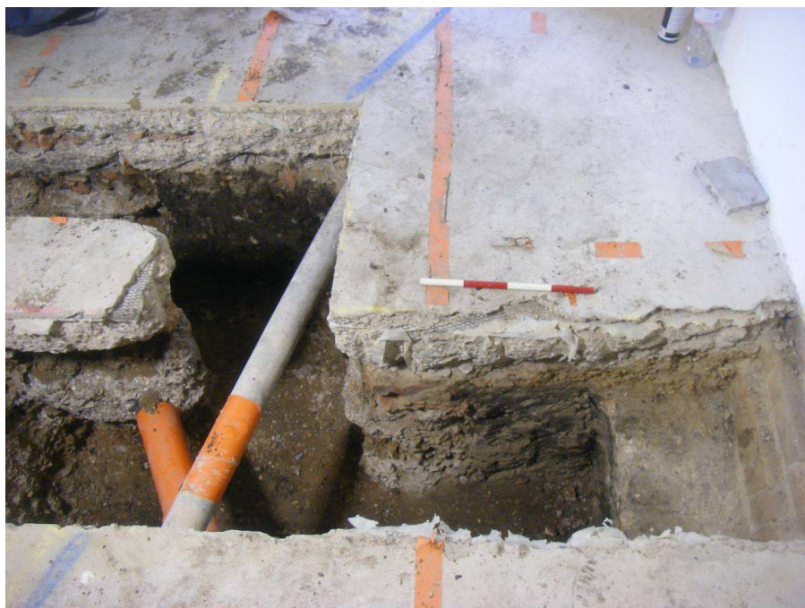
Image 1: Eastern end of Trench 1 looking north (scale 40cm)
