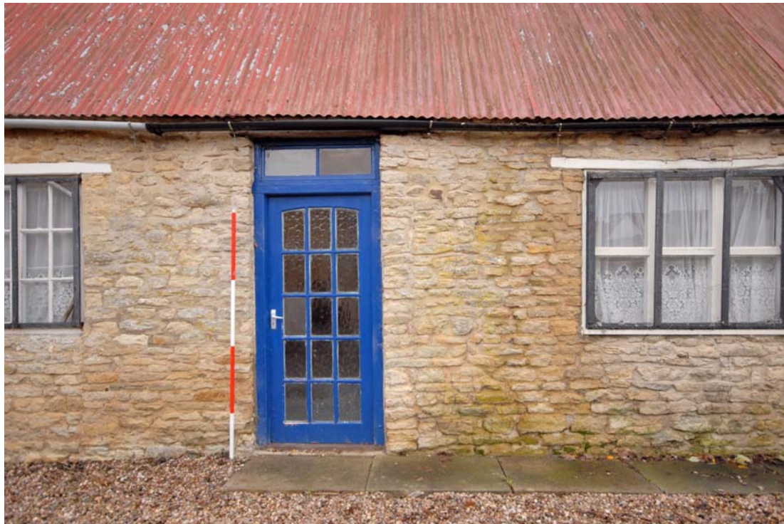
Image 12: Exterior: central section of west elevation
