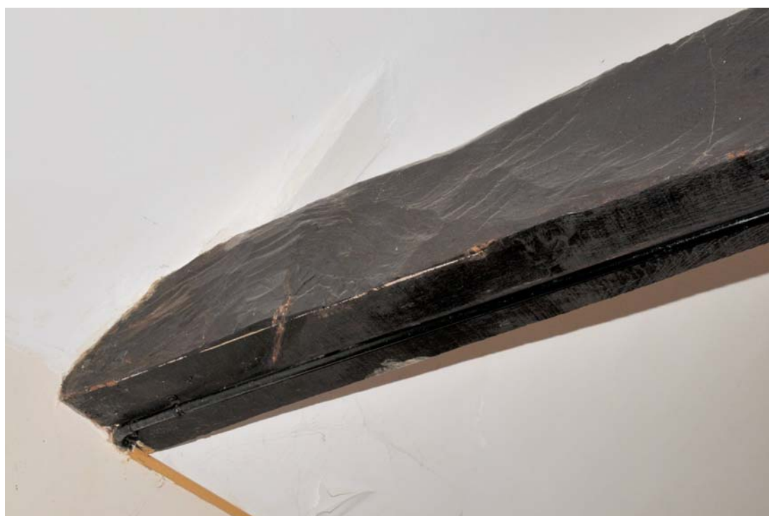
Image 18: Interior: detail of east end of northern tie beam View looking south east showing roughly hewn north side
