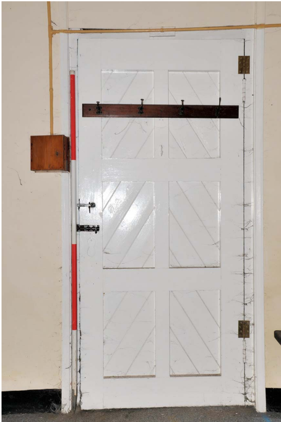
Image 19: Interior: south door Showing internal framing and diagonal plank covering
