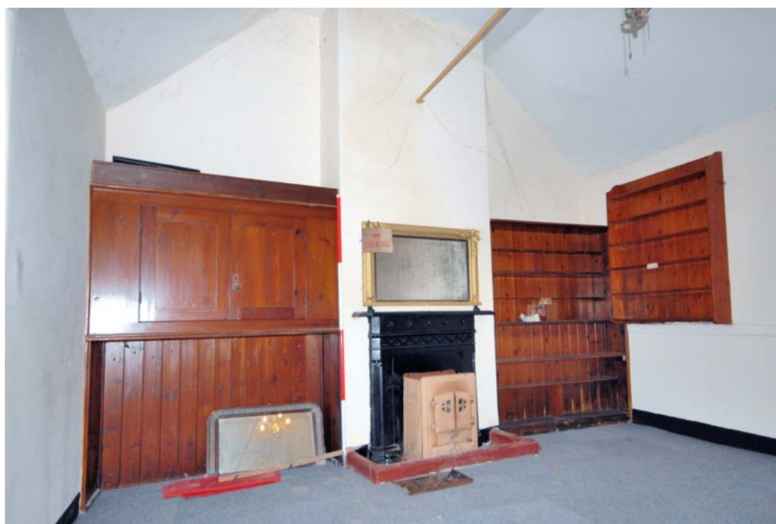
Image 27: Interior detail at north end of room
