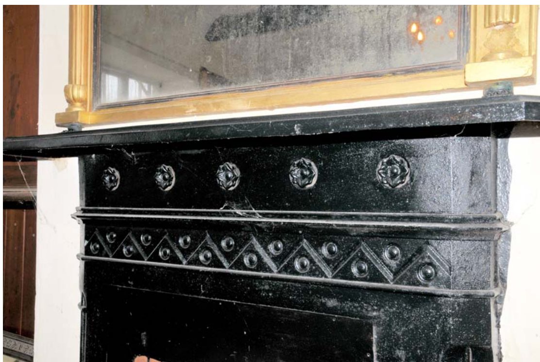
Image 21: Interior: detail of fireplace
