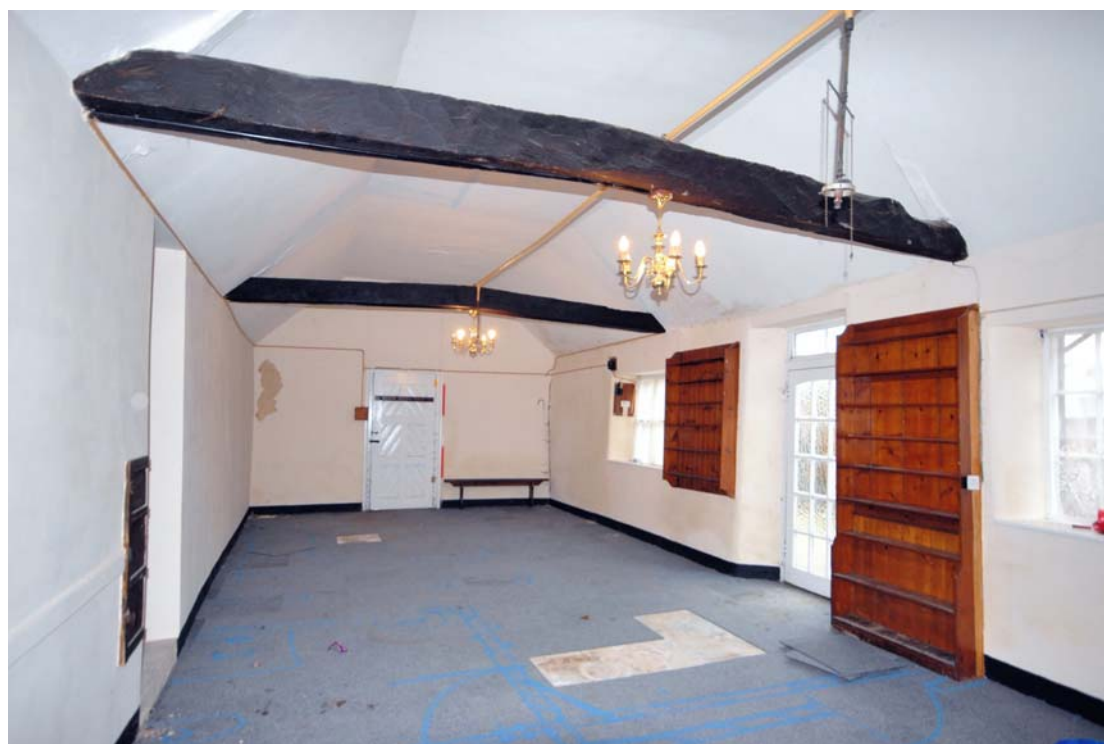
Image 14: Interior looking south west
