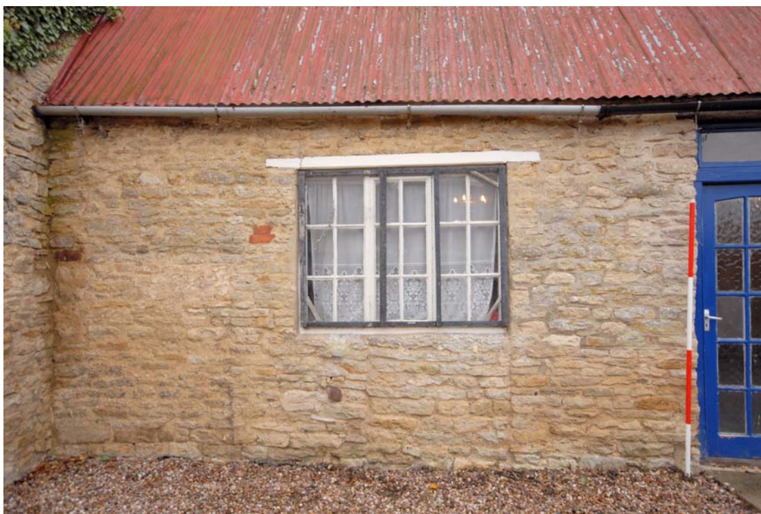
Image 11: Exterior: northern end of west elevation
