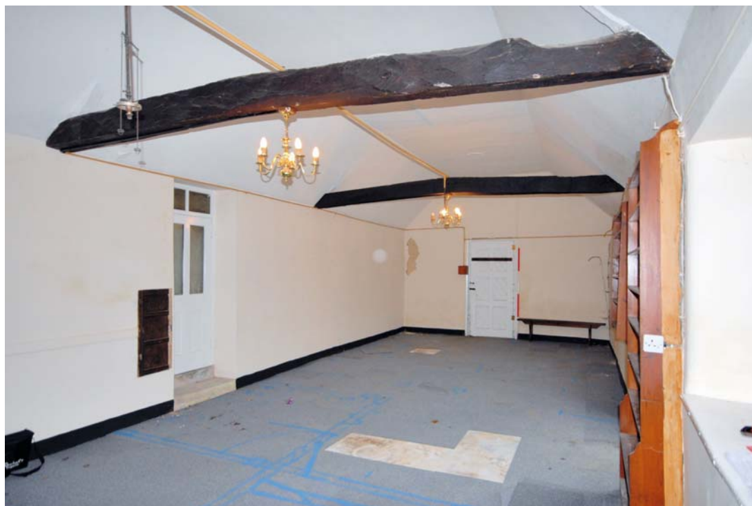
Image 15: Interior looking south east
