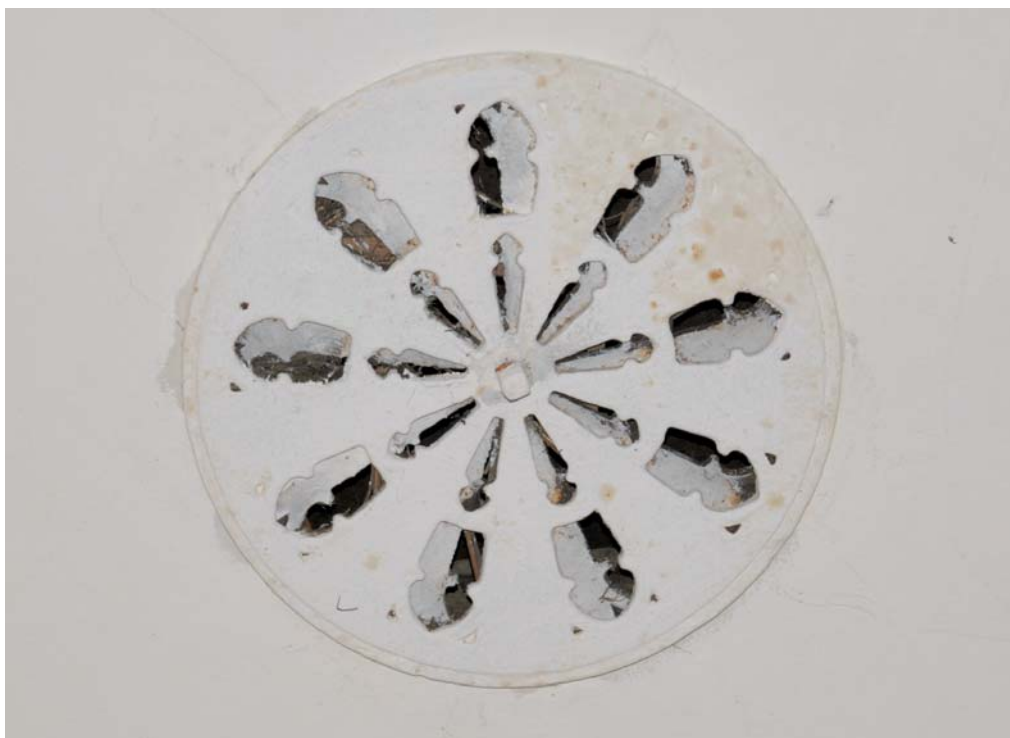
Image 24: Interior: detail of ceiling vent
