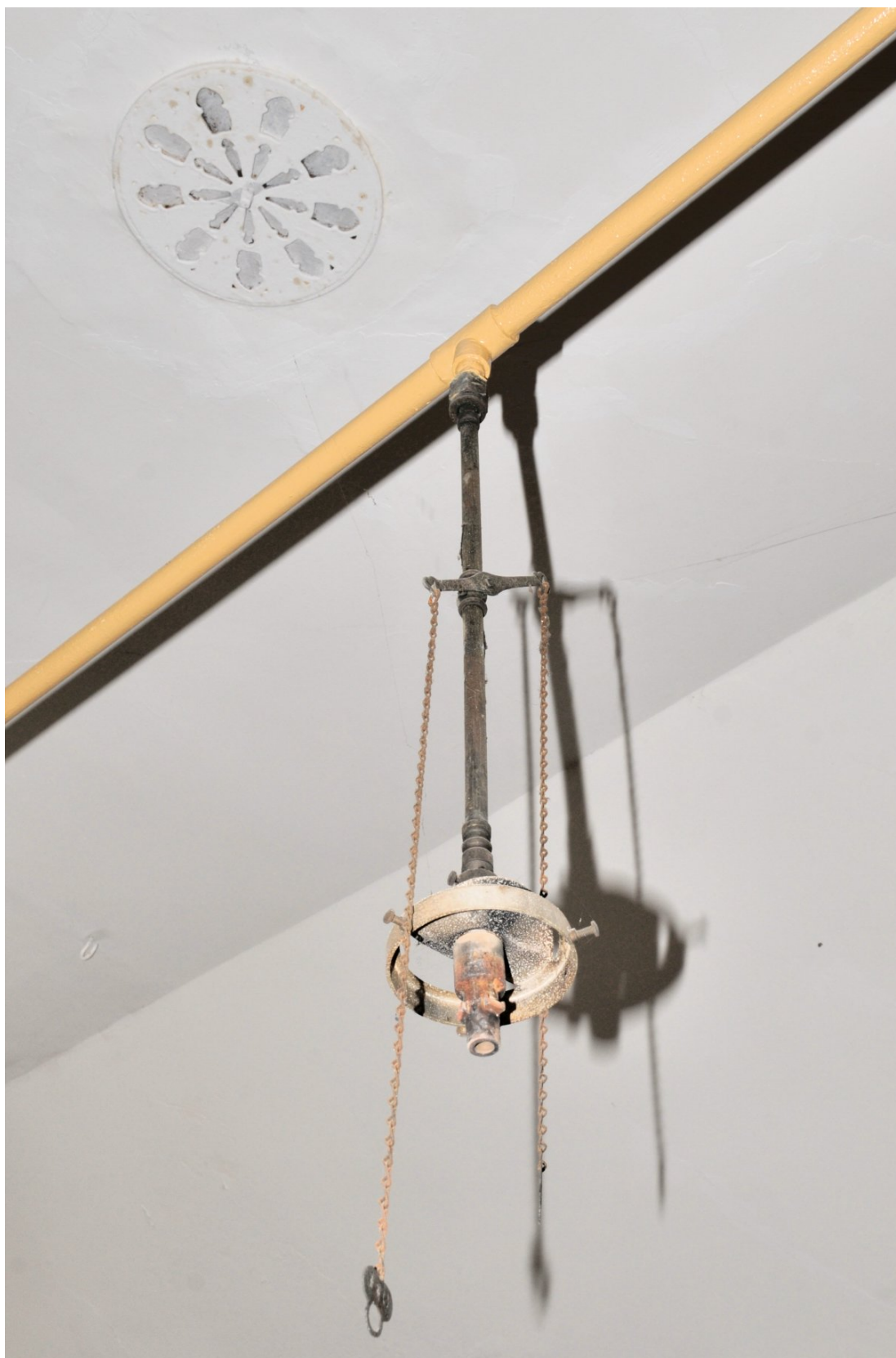
Image 23: Interior: detail of gas light fitting
