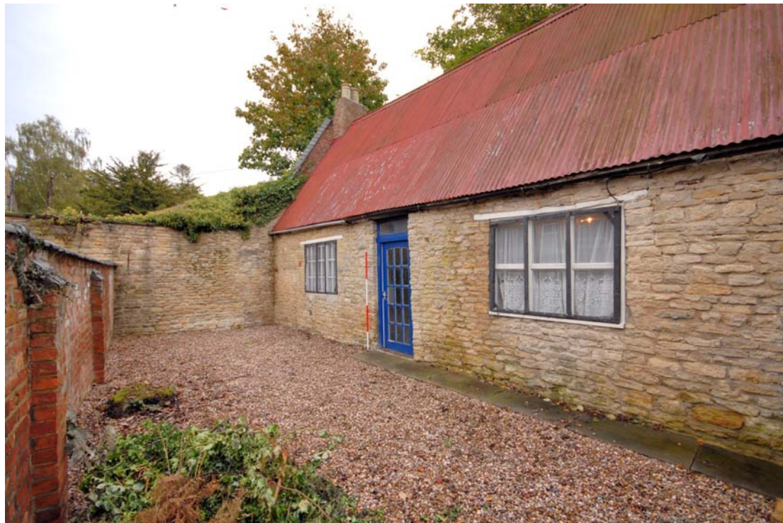
Image 10: Exterior from the south west showing west elevation
