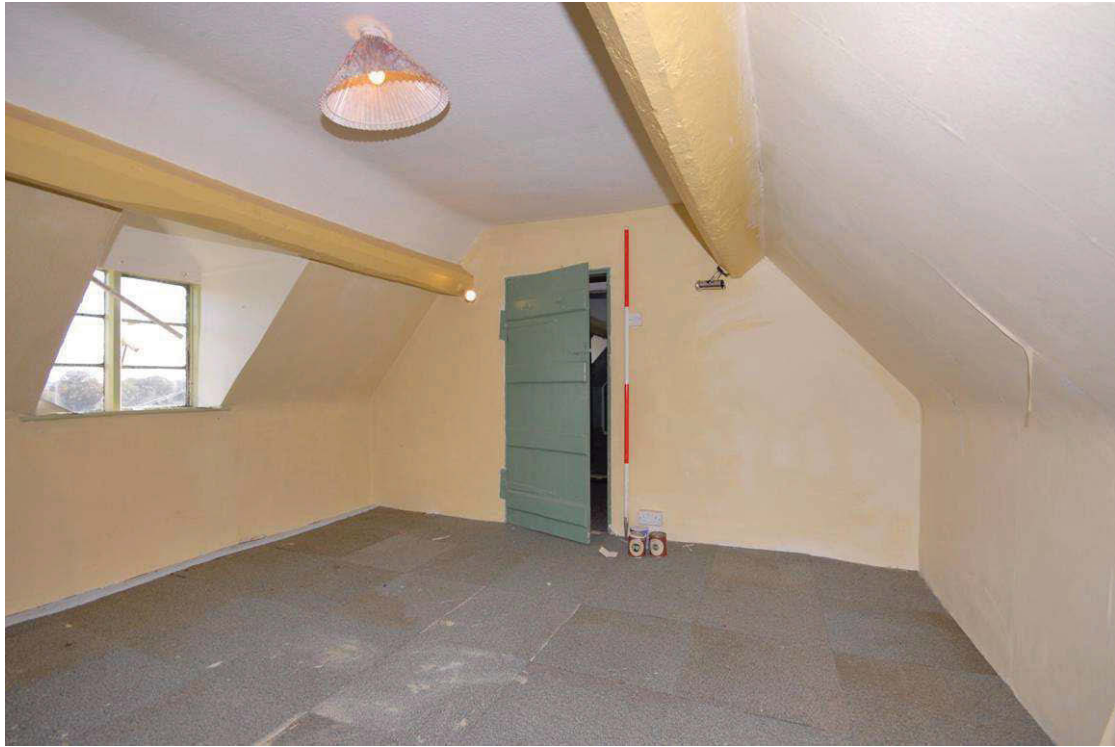
Image 39: Second floor room 2 Looking south east
