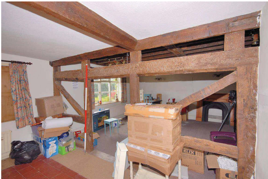
Image 18: Ground floor room 4: detail of timber partition Looking south west
