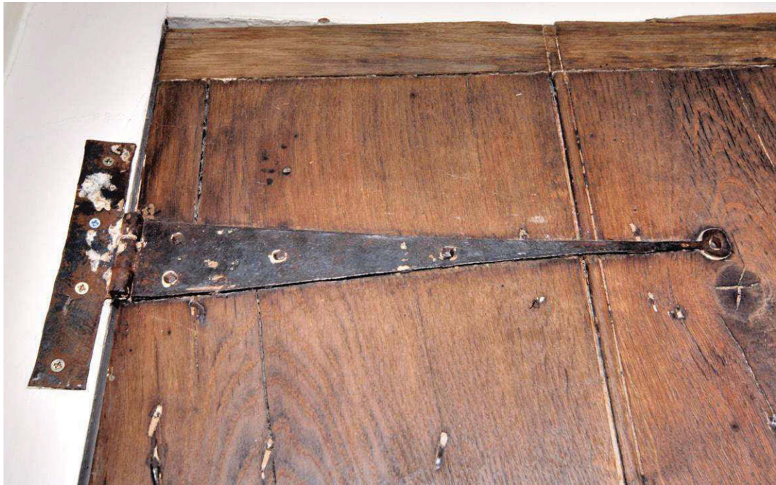
Image 35: First floor land: detail of stair door H-shaped hinge with rounded terminal
