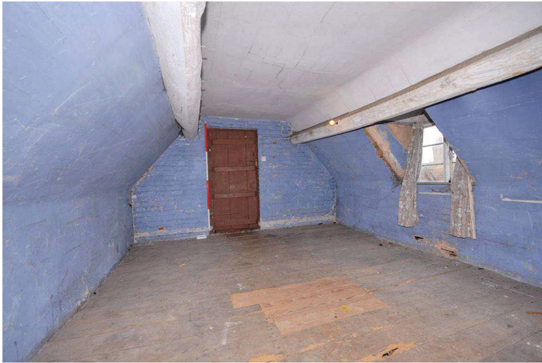
Image 37: Second floor room 1 Looking south
