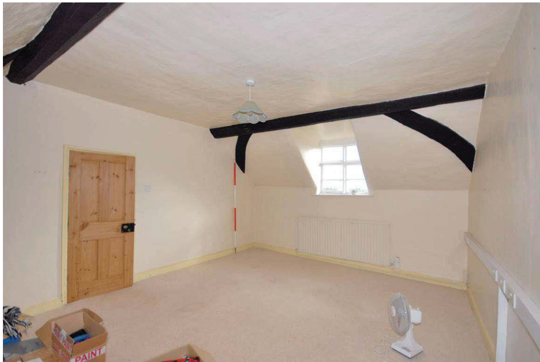
Image 29: First floor room 4 Looking south east
