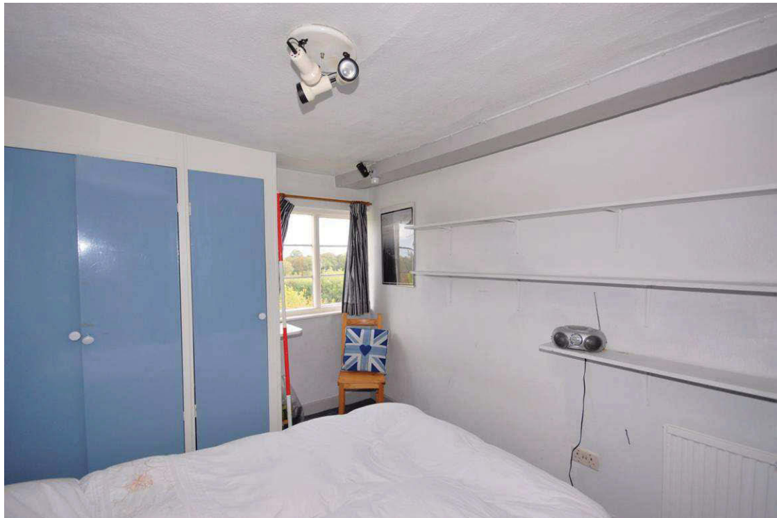
Image 27: First floor room 2 Looking south east showing modern partition wall just beyond beam
