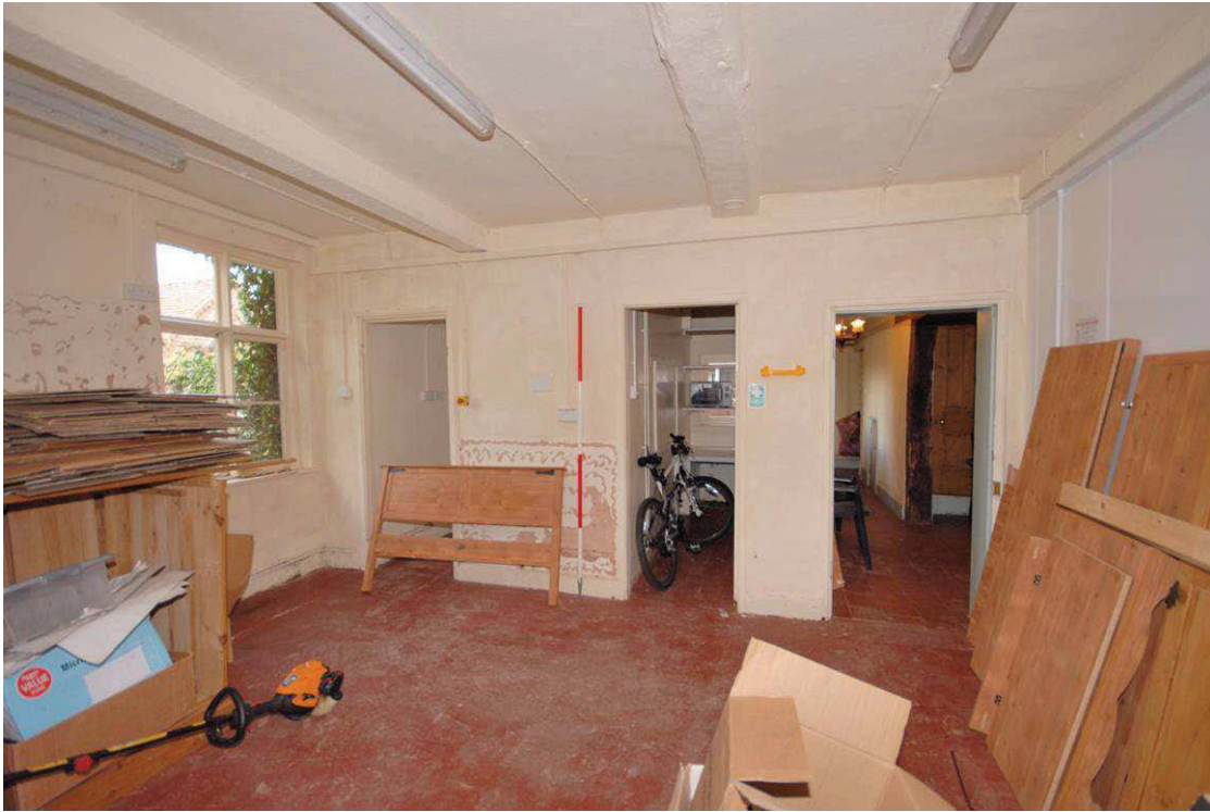
Image 21: Ground floor room 6 Looking east, towards the lobby, larder and corridor
