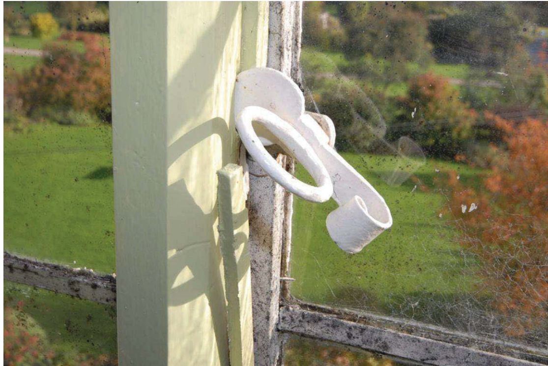
Image 40: Second floor room 2: detail of window catch
