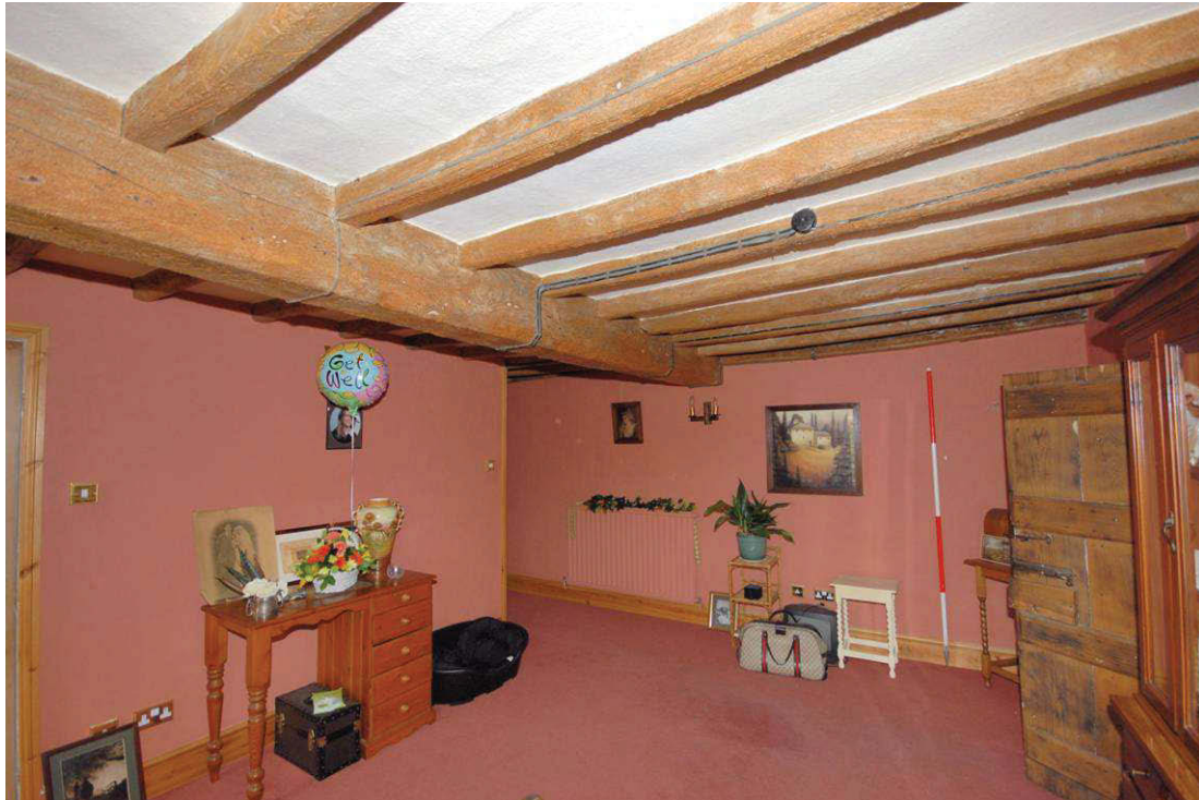
Image 12: Ground floor room 2 Looking south west
