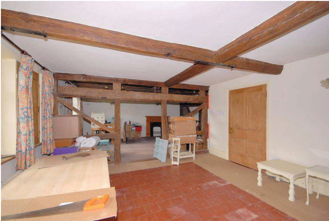
Image 17: Ground floor room 4 Looking north west
