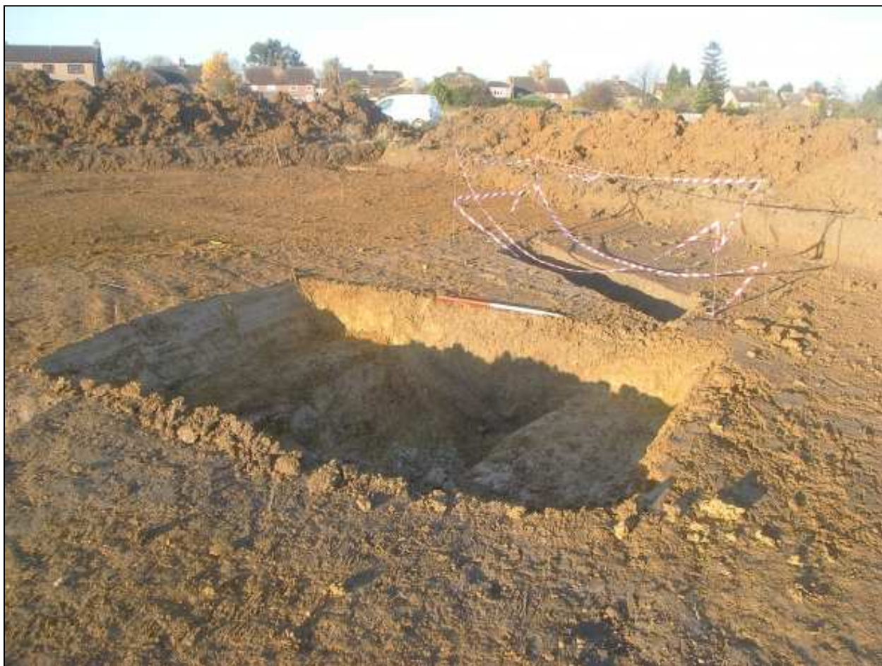
Figure 4: Photograph of machine-excavated ditch segment [1239] with original segment [303] in background
