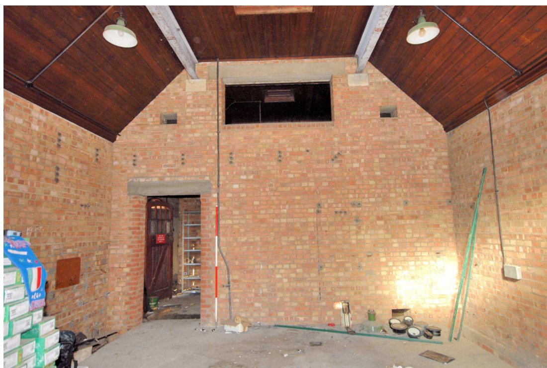
Image 16: Interior: North wall of south room Facing north (scale 2m)
