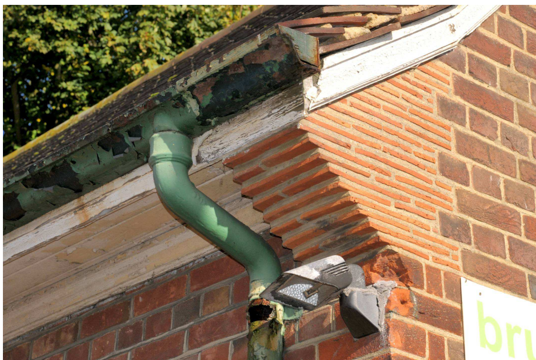
Image 10: Exterior detail: Tile corbel and eaves Image shows south west corner of building. View facing north east
