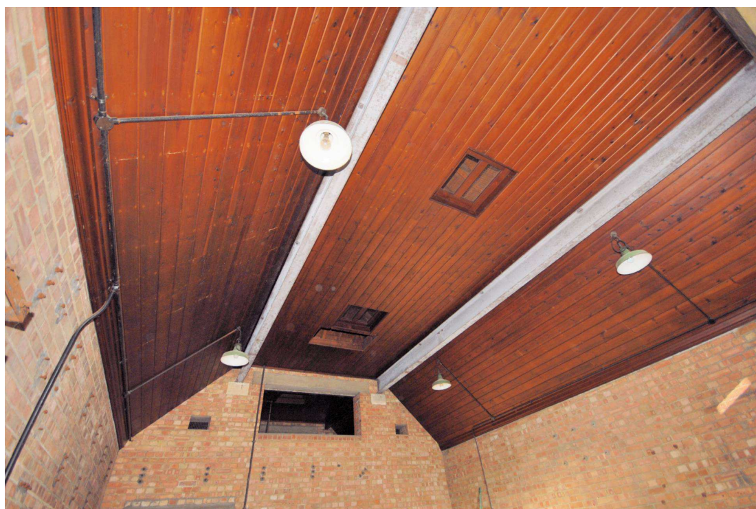
Image 18: Ceiling of south room Facing north, north east
