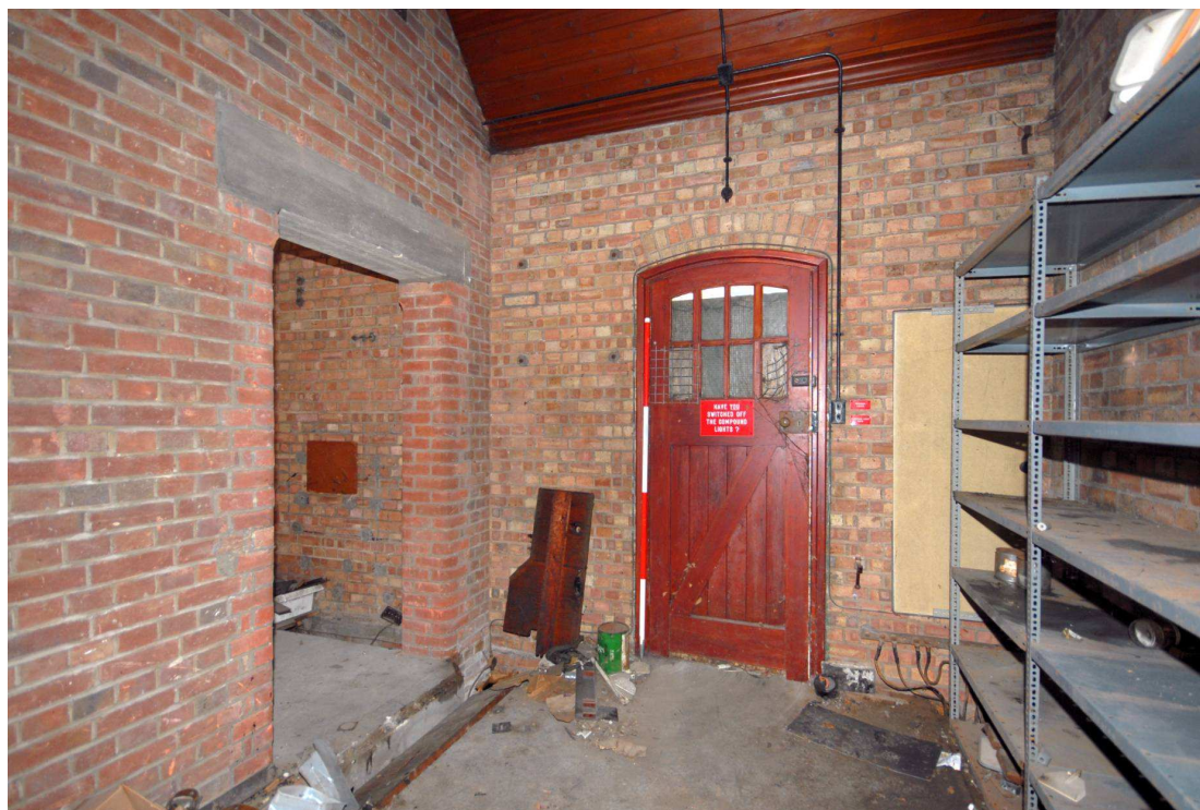
Image 21: Interior: West wall of north room Facing south east (scale 2m)
