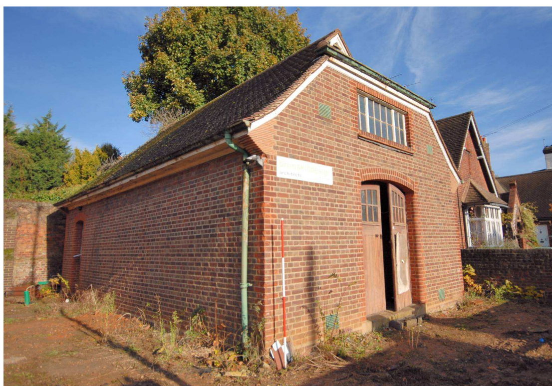
Image 8: Exterior showing south and west elevations Facing north east (scale 2m)
