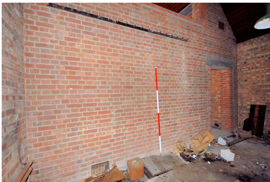
Image 20: Interior: South wall of north room Facing south west (2m scale)
