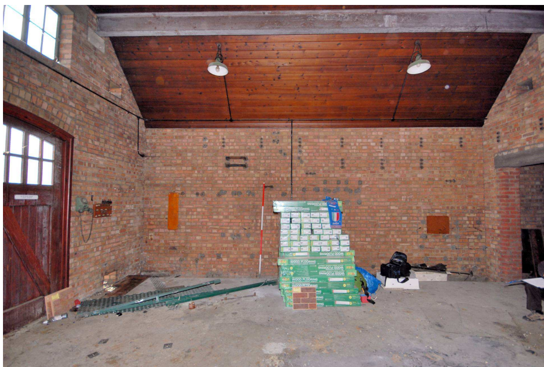
Image 15: Interior: West wall of south room Facing west (scale 2m)
