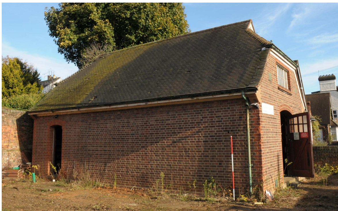
Image 7: Exterior showing west elevation Facing east, north east (scale 2m)
