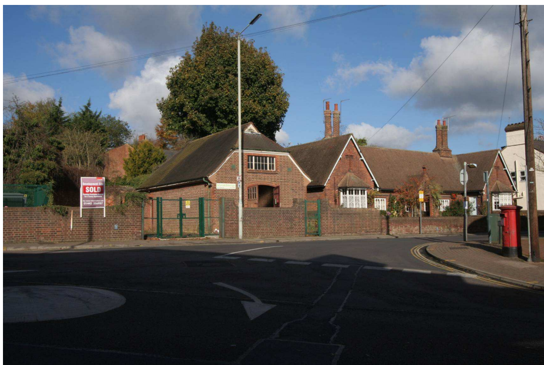
Image 6: View of the substation looking north
