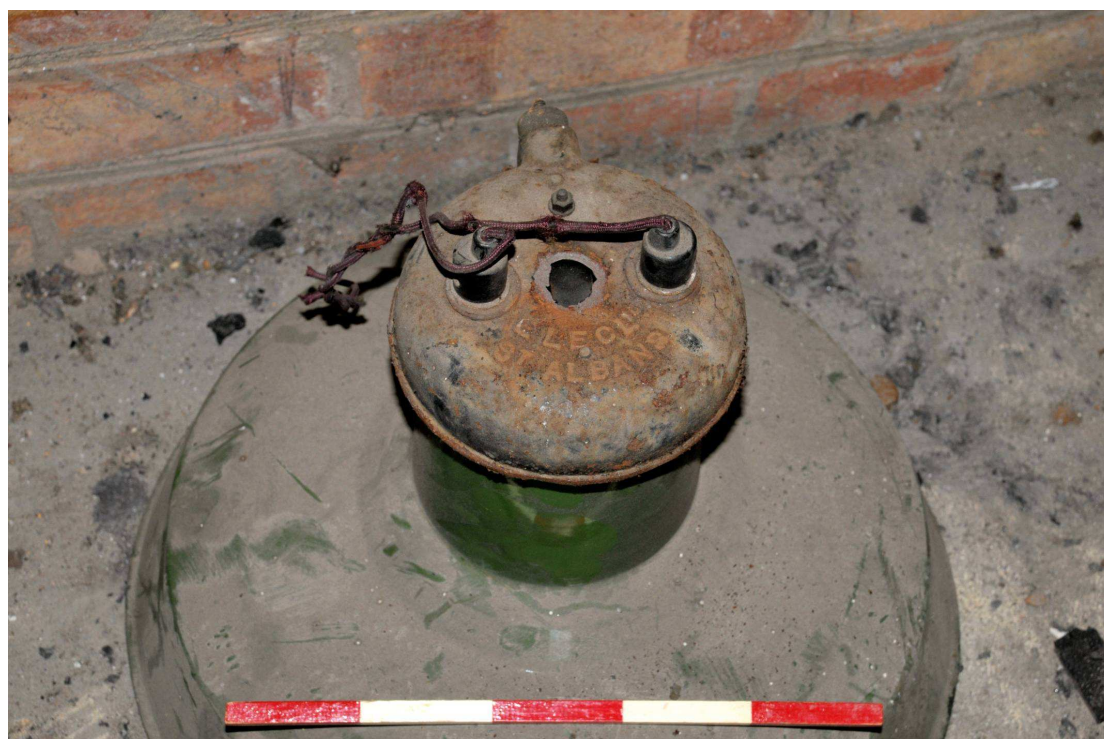
Image 24: Interior detail: Light fitting Top of light carries name ELEC L td ST ALBANS (scale 25cm)
