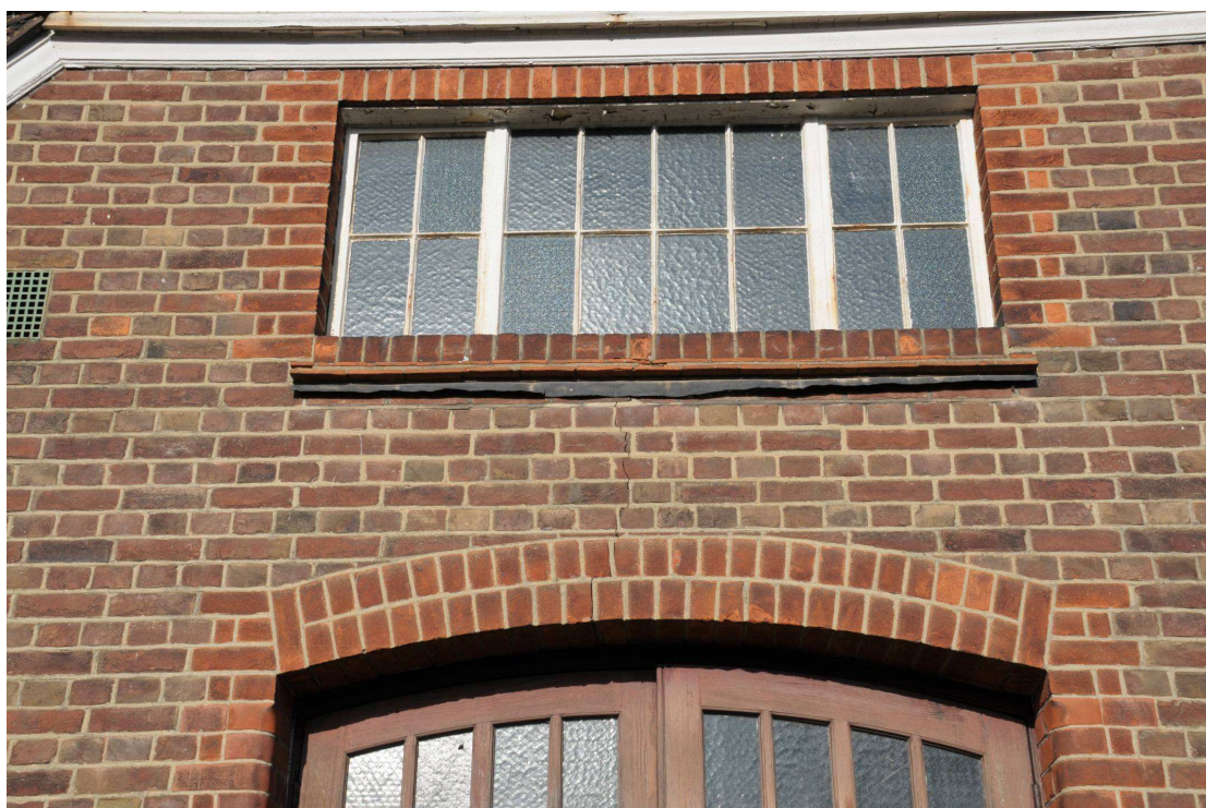
Image 12: Exterior detail: Window in south elevation
