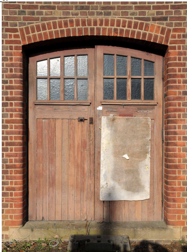
Image 13: Exterior detail: Door in south elevation
