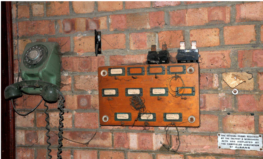
Image 26: Interior detail: Fittings on south wall of main room
