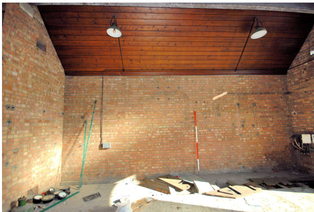
Image 17: Interior: East wall of south room Facing east (scale 2m)
