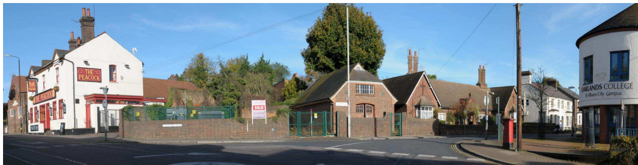
Image 5: Substation and nearby buildings Composite panoramic view looking north
