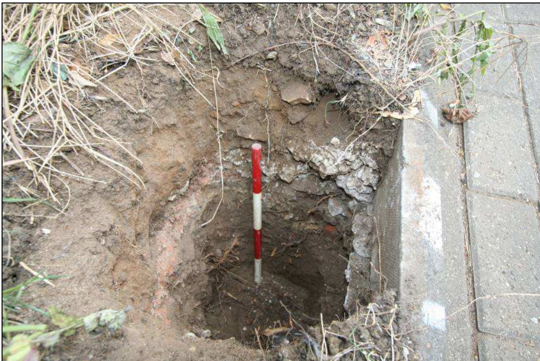
Image 6: Amenity area fencing Showing typical posthole for fence adjacent to pavement on St John's Street, looking north (40cm scale)
