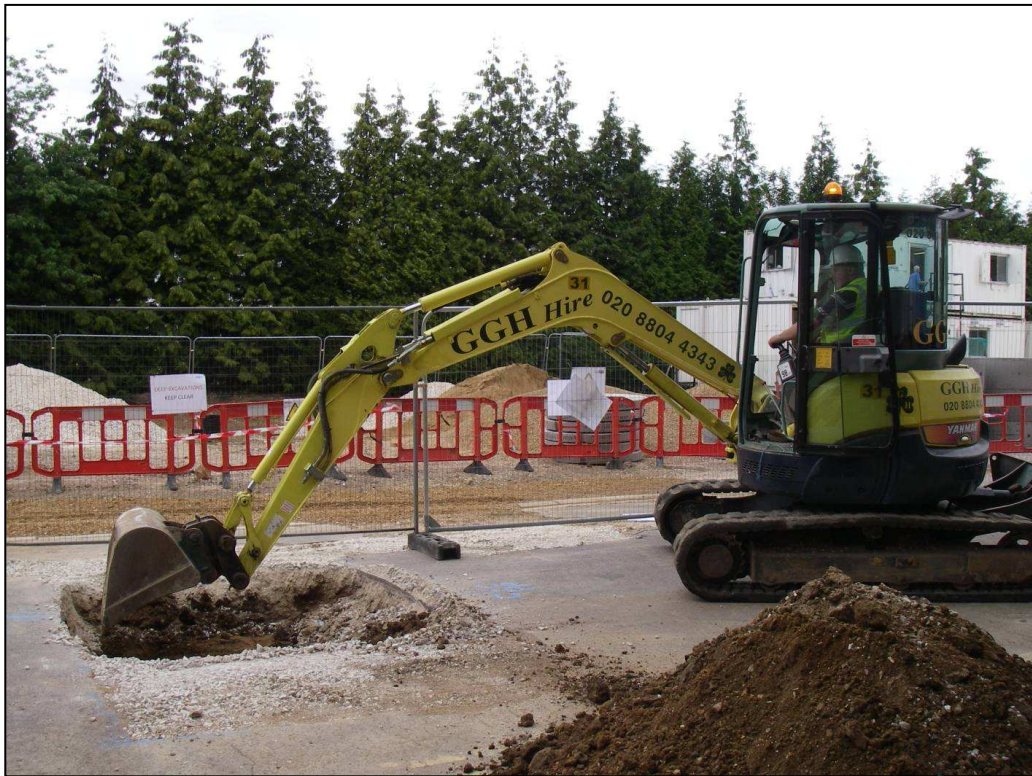
Image 2: Trench 7 (inspection chamber) Machine excavation
