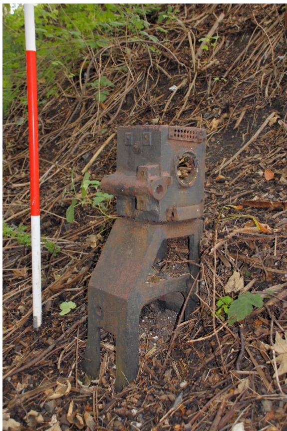
Plate 22: Ground signal (old) west of Crawley Green Bridge
