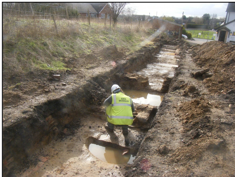
Ironstone wall footings
