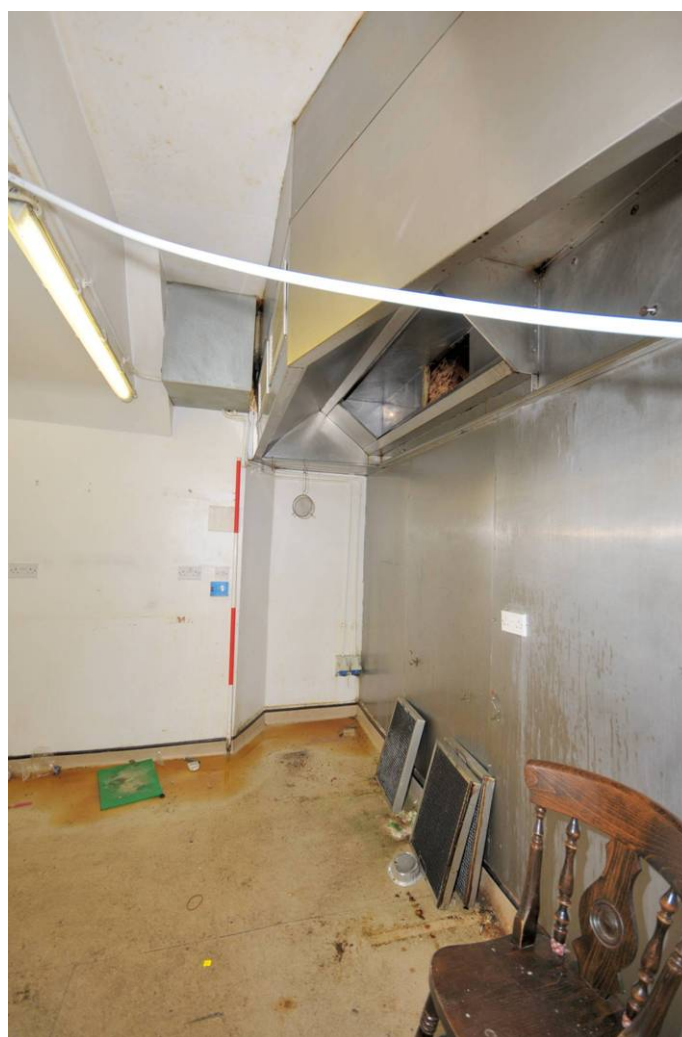
Plate 14: Kitchen showing splayed wall between lean-to and main structure
