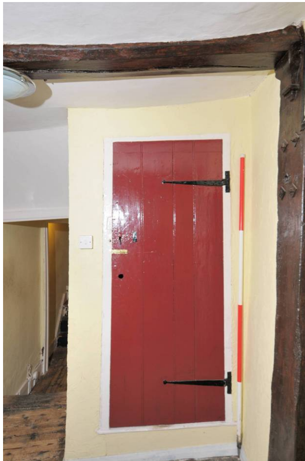
Plate 21: Main range, first floor, north room, attic stair door
