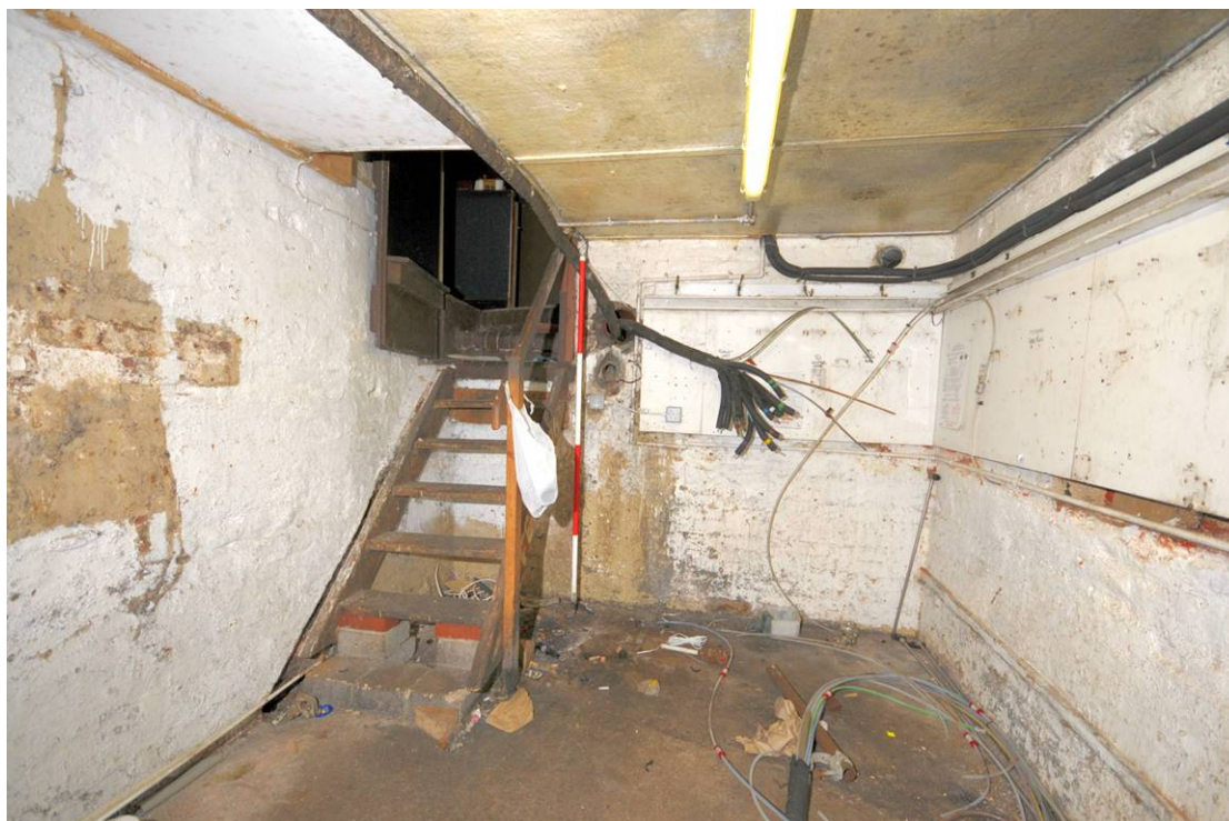
Plate 5: Cellar looking west
