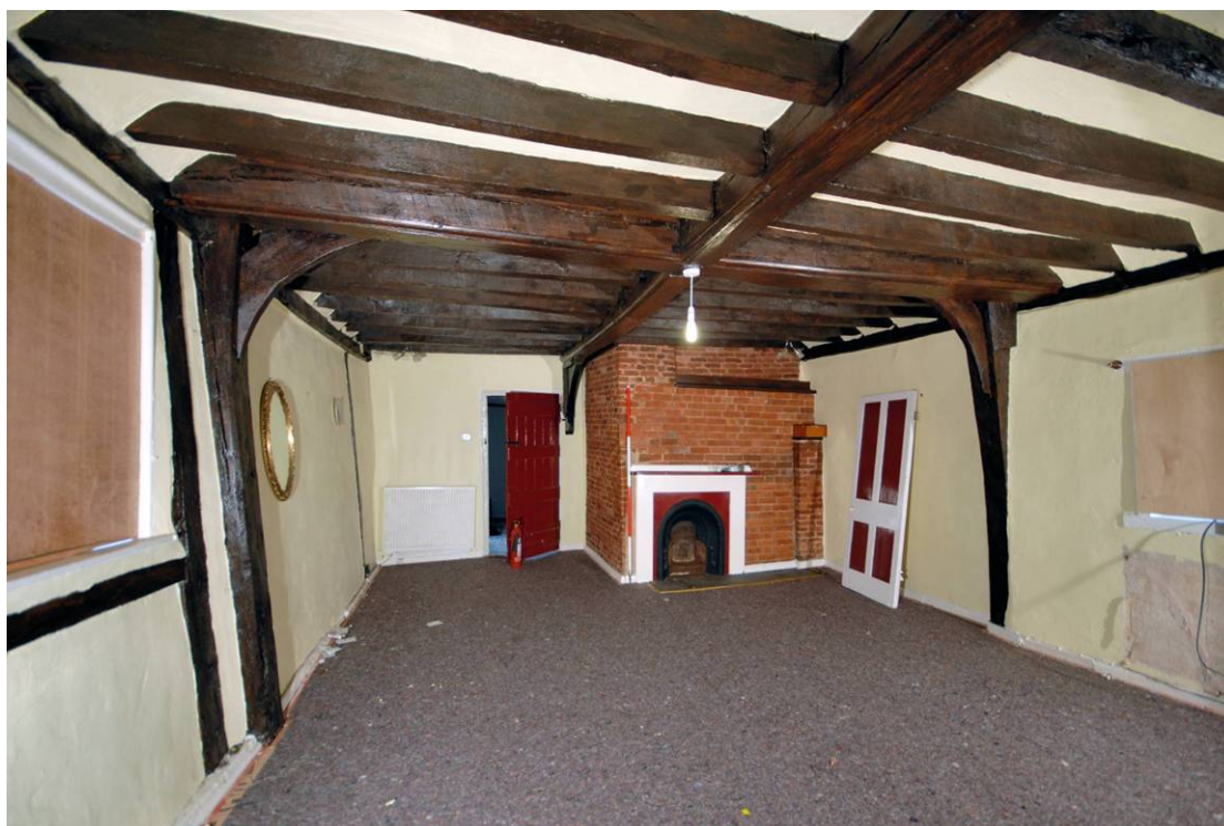
Plate 16: Main range, first floor, south room looking north Shows original stack with inserted Victorian fireplace and inserted ceiling with ovolo chamfered beams.
