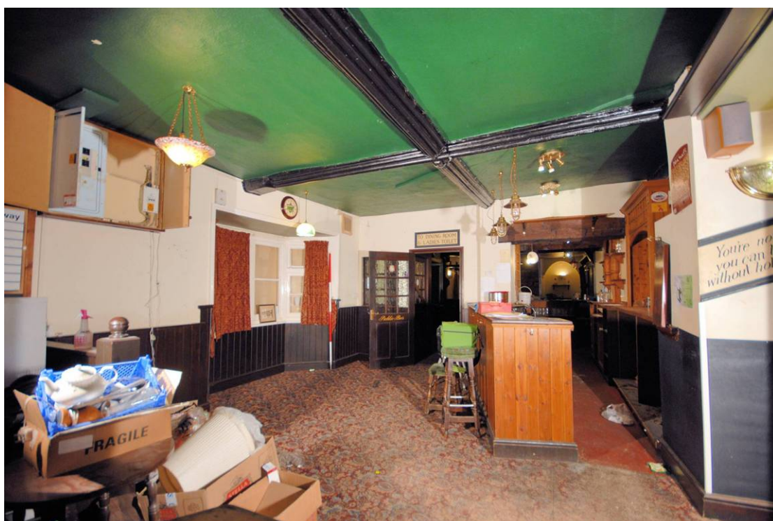
Plate 6: Main range, ground floor looking north from south end
