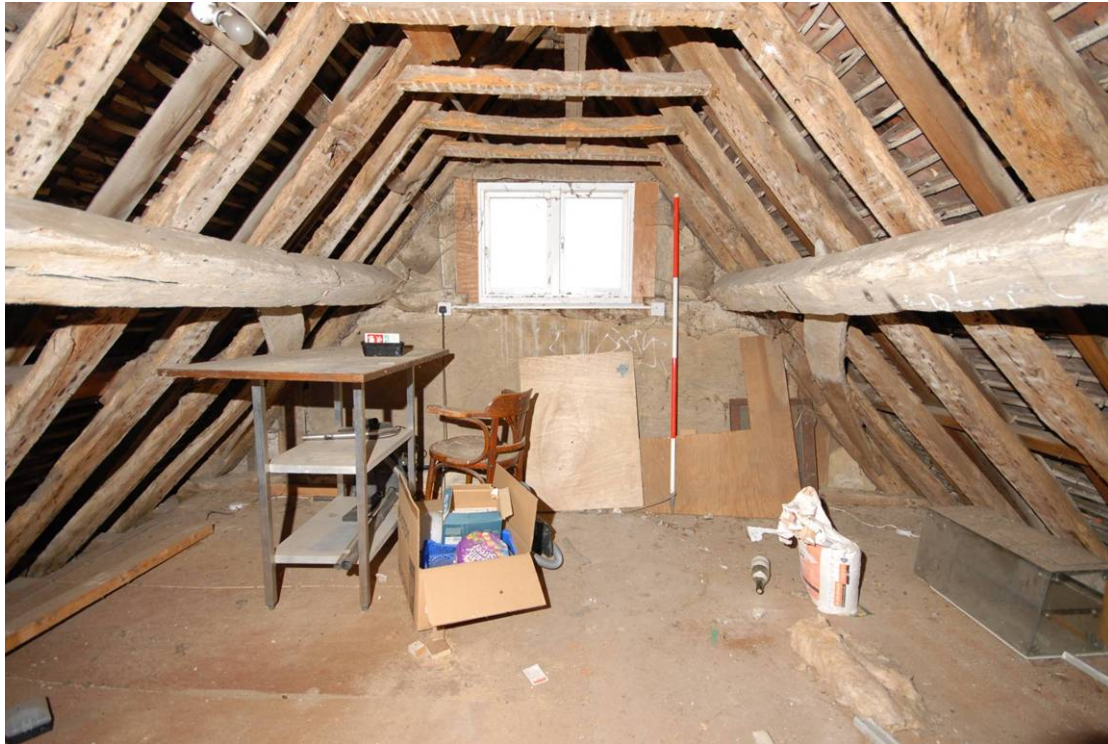
Plate 23: Main range, attic, south bay, looking south
