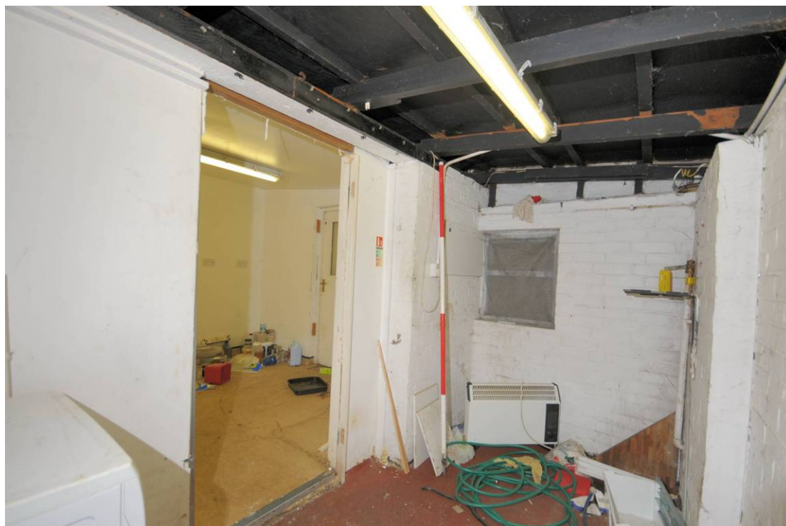
Plate 15: Modern extension on east side of rear wing
