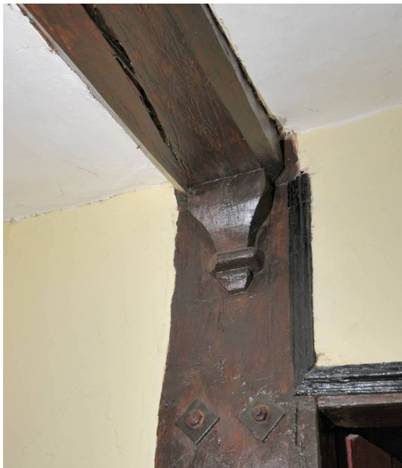
Plate 20: Main range, first floor, north room, chamfered beam and pendant Pendant at south end of plain chamfered axial ceiling beam.
