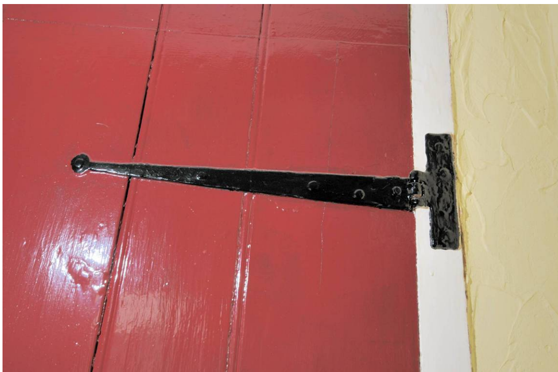
Plate 22: Detail showing hinge on attic stair door
