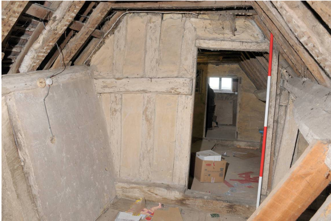
Plate 29: Main range, attic, north bay, looking south Shows close studded bay division with inserted doorway
