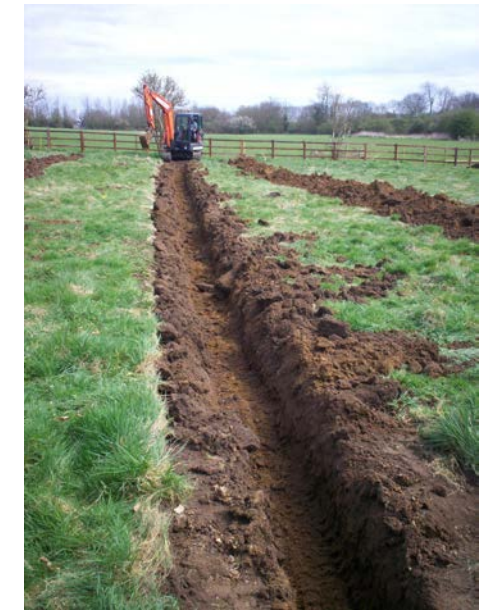
Southern land drain trench
