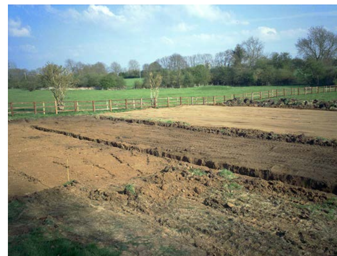
Southern half of stripped area showing subsoil and topsoil
