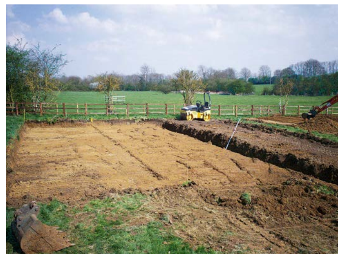
Northern half of stripped area showing subsoil and Boulder Clay
