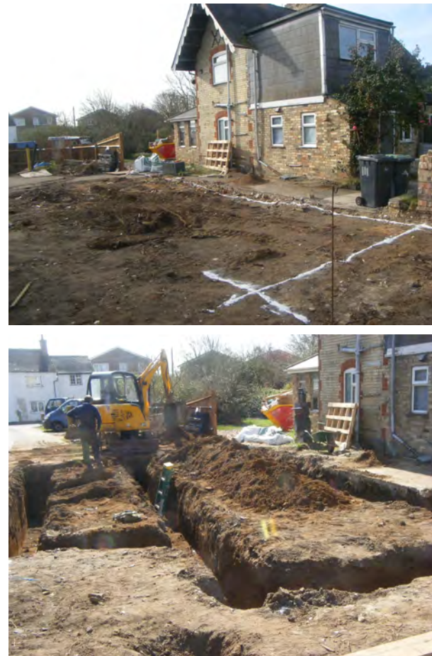
General views before and after machining
