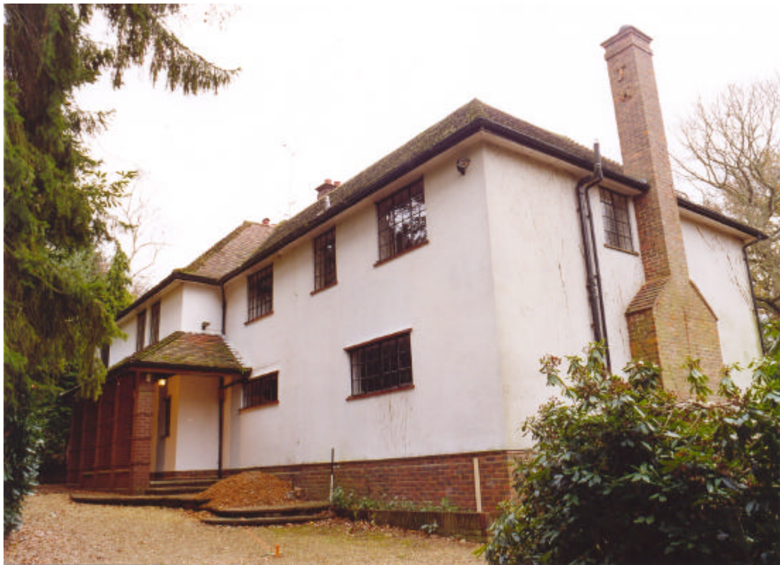
Plate 1b: External View showing frontage (view east-south-east)
