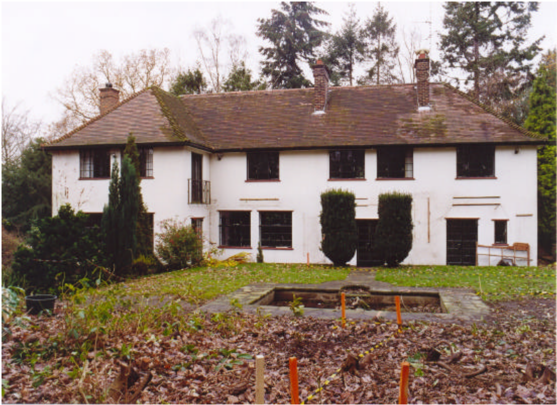
Plate 1a: External Elevation (view north)
