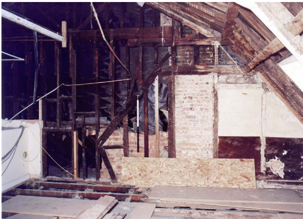
Plate 24: Attic floor, southeast corner, showing framing of 18 th century gable incorporated into 19 th century mansard roof structure
