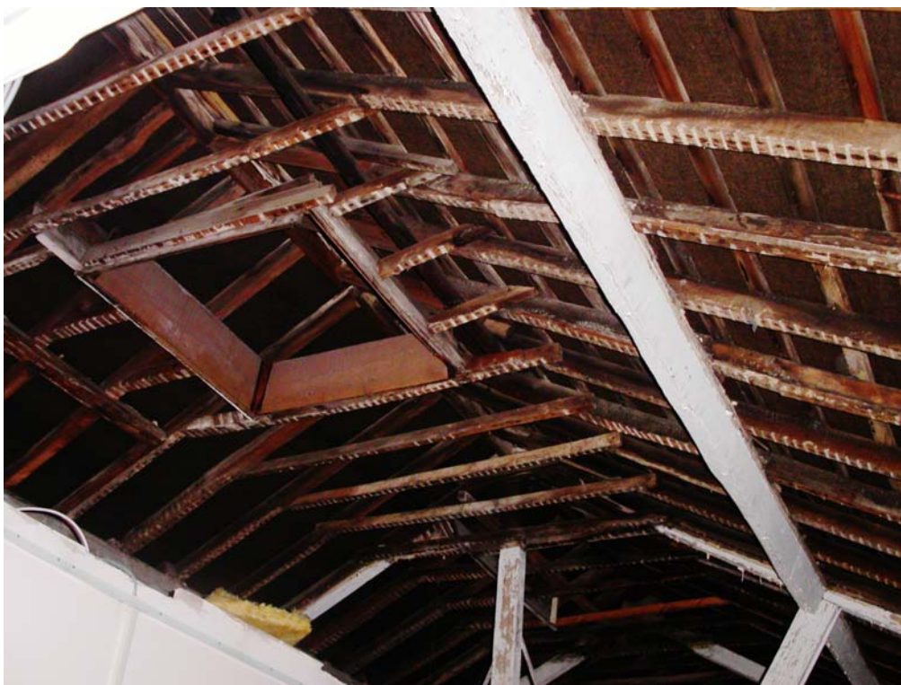
Plate 25: Attic floor, roof structure, showing framing of former ventilator
