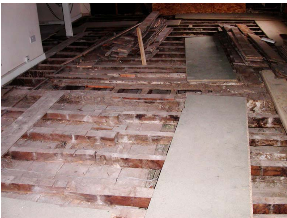
Plate 26: Attic floor, showing earlier floorboards preserved beneath later floor level
