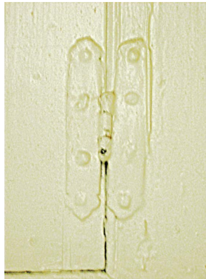
Plate 18: First floor, H-shaped hinge on cupboard
