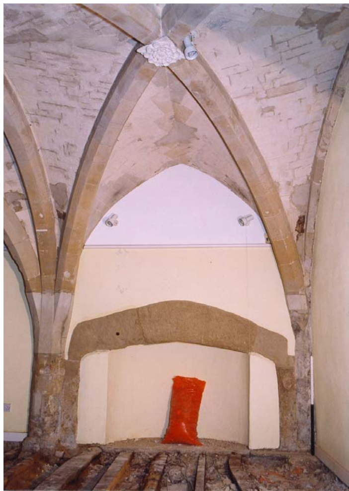
Plate 9: Ground floor, Room G1 reconstructed fireplace in northeast corner of room
