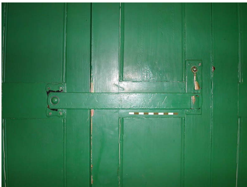
Plate 20: Shutter closure (scale 10cm)
