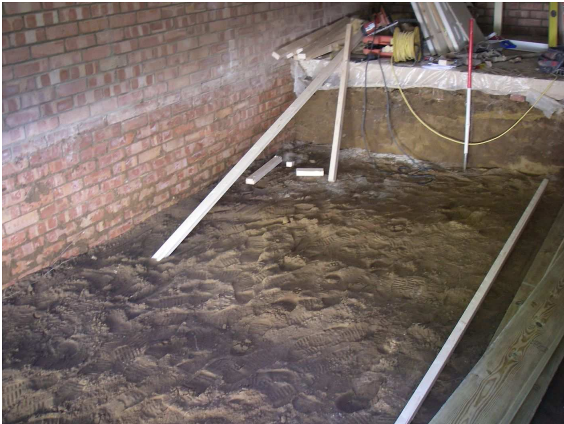
Figure 5: Ground reduction within garage
