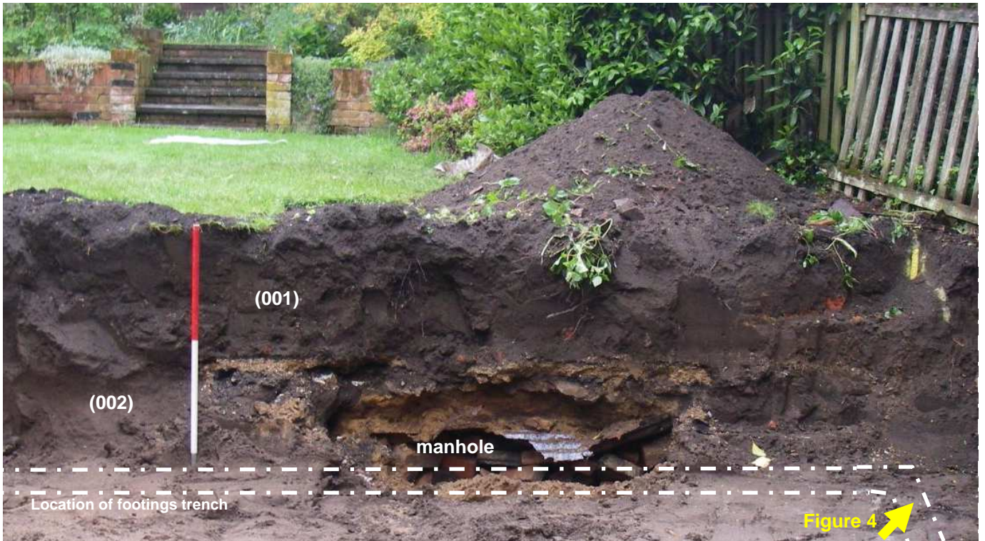
Figure 3: Ground reduction prior to construction of footings
