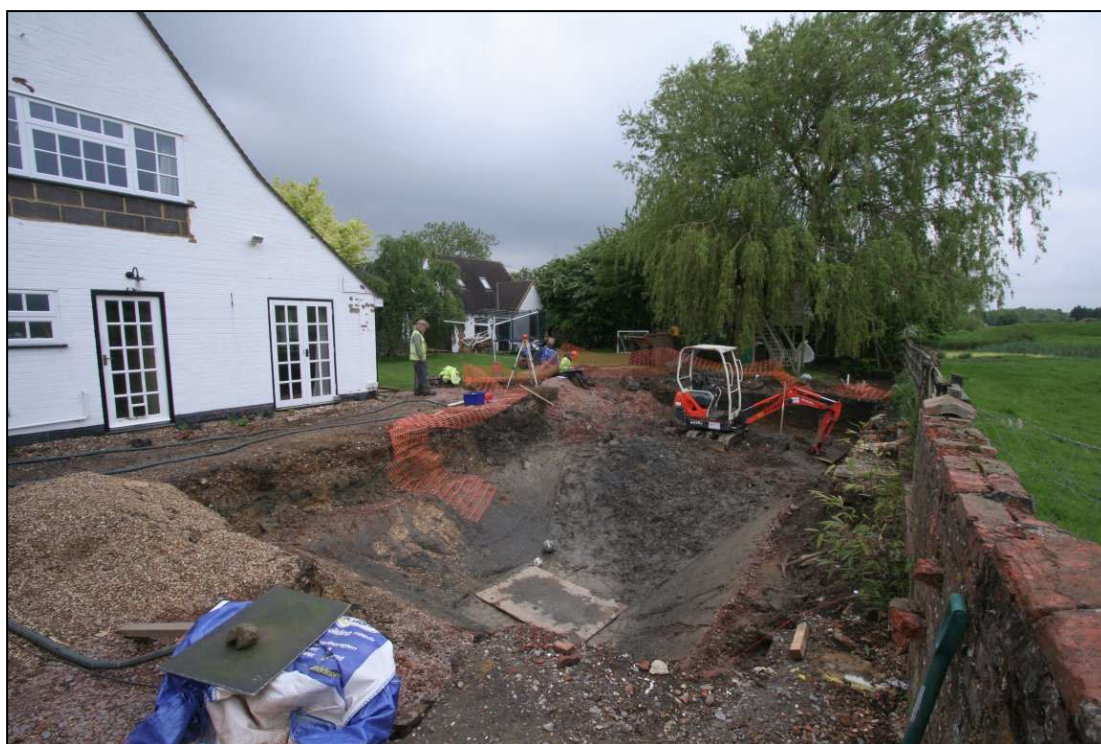
Plate 2: View of trench looking north-west
