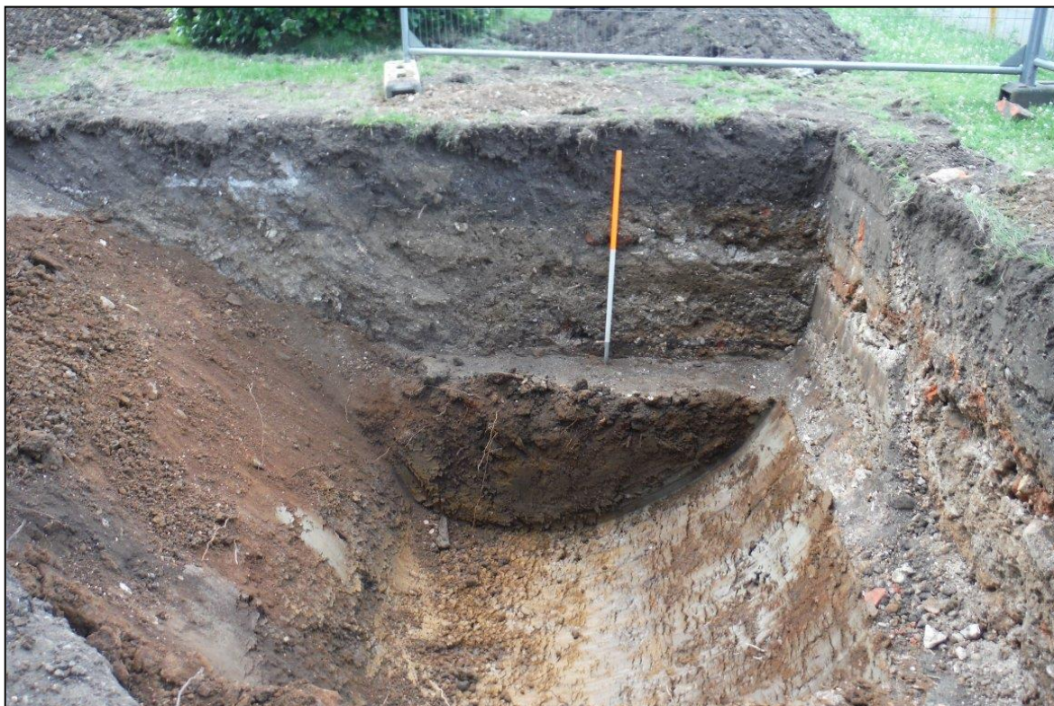
Image 6: Trench 1, machine-excavated section
