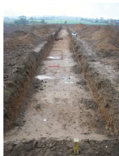
Trench 4 looking north-east
