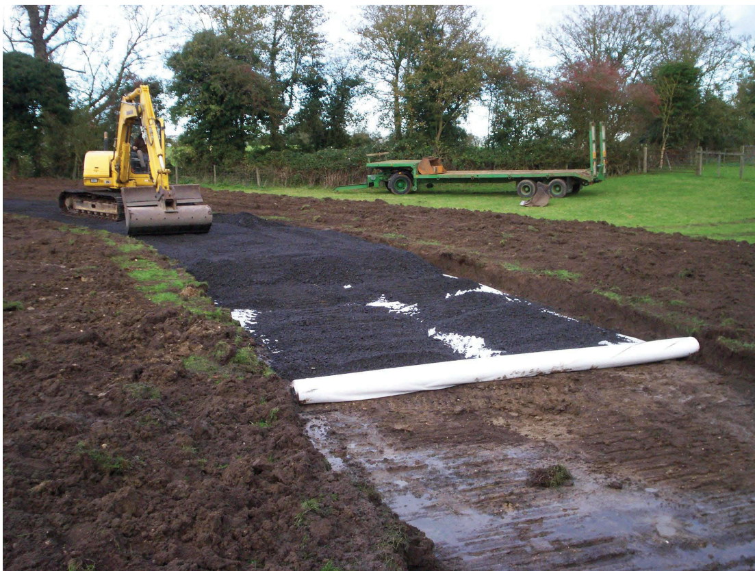
Figure 4: Access track with covering membrane and hardcore
