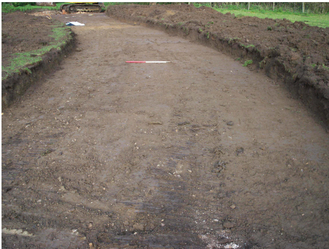
Figure 3: Central part of access track after machining looking NNW
