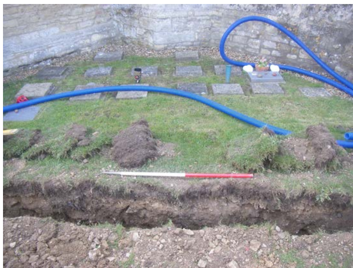
Image 7: Water pipe trench north-west of tower looking south-east (scale 1m)
