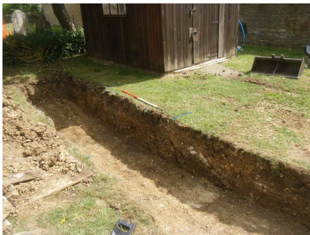
Image 11: Trench-arch 2, south of church looking south-east (1m scale)
