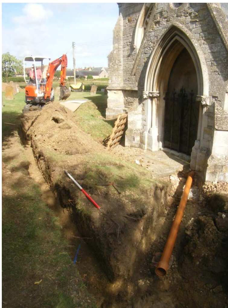
Image 8: Water pipe trench in front of south porch (1m scale)
