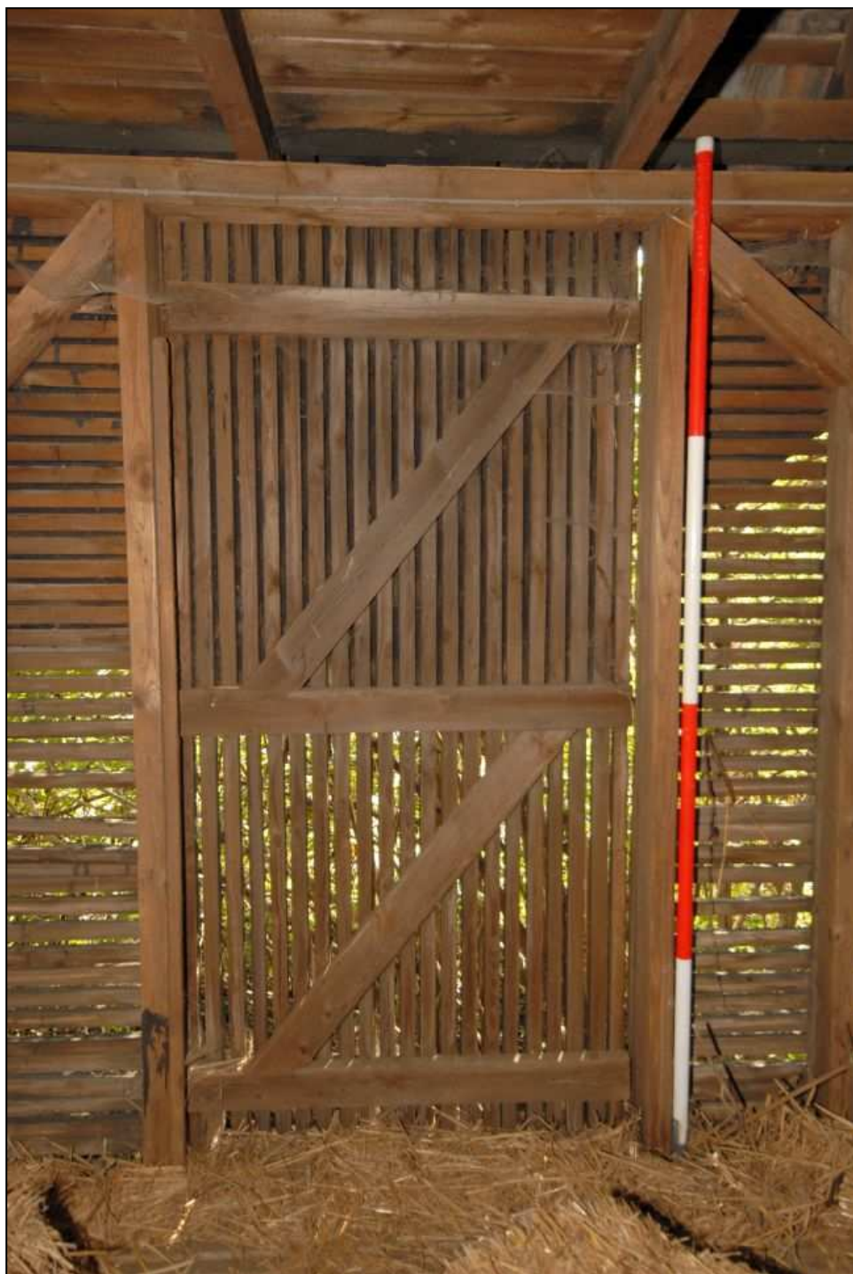
Image 11: Interior view showing door in east side wall (scale 2m)
