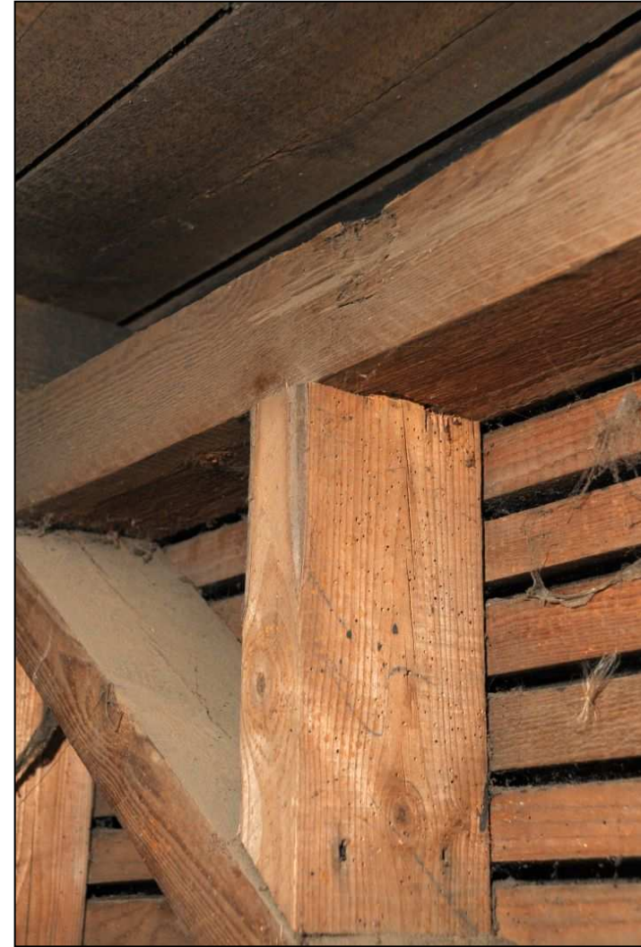
Image 15: Interior detail showing upper part of west side wall
