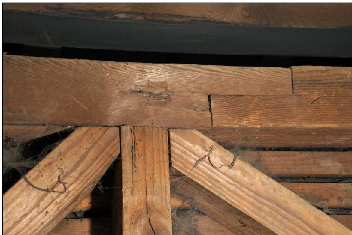
Image 13: Interior detail of west wall showing scarf joint in wall plate
