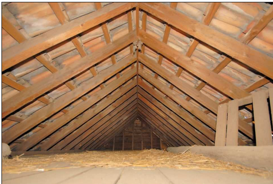
Image 12: Interior view showing loft and roof structure
