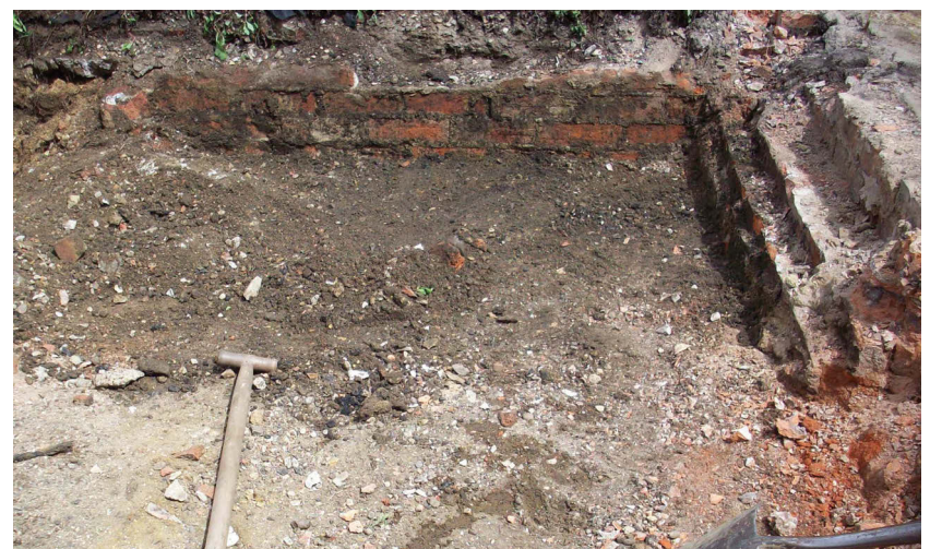
Remains of previous foundations in SE corner of site
